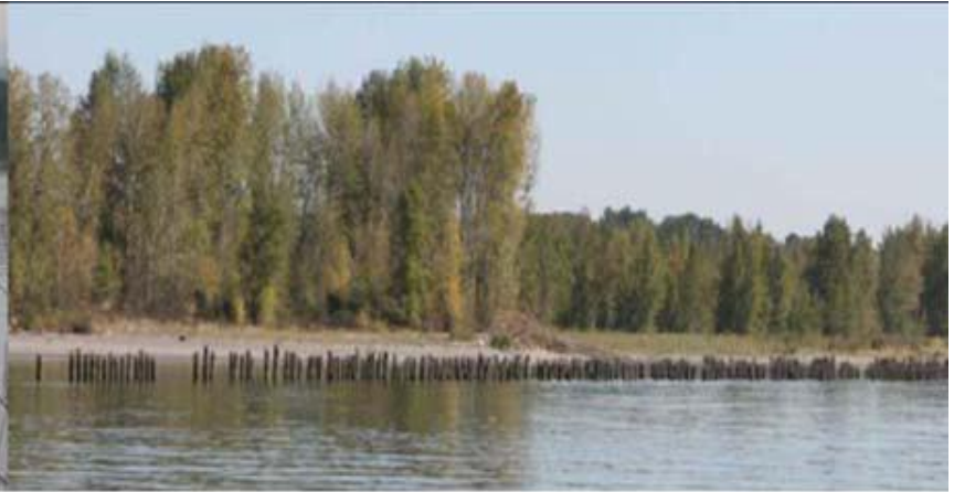
Training Pile Dike
