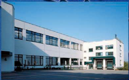
Production facility in Wetter-Volmarstein
