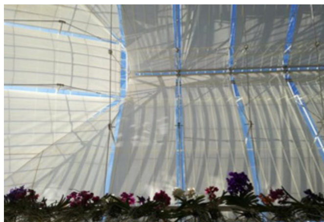
Figure 5: Automated ceiling screens
