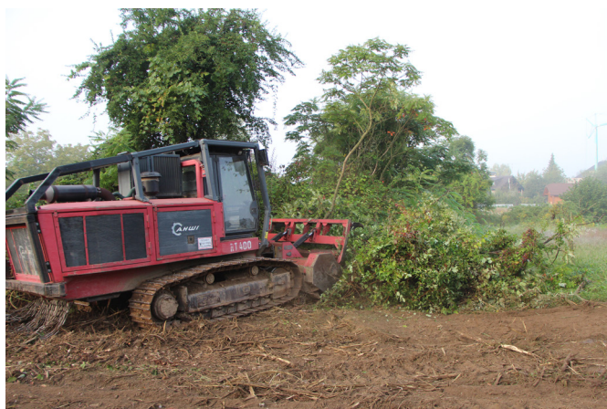
Figure 1: Cleaning the area with a mulcher
