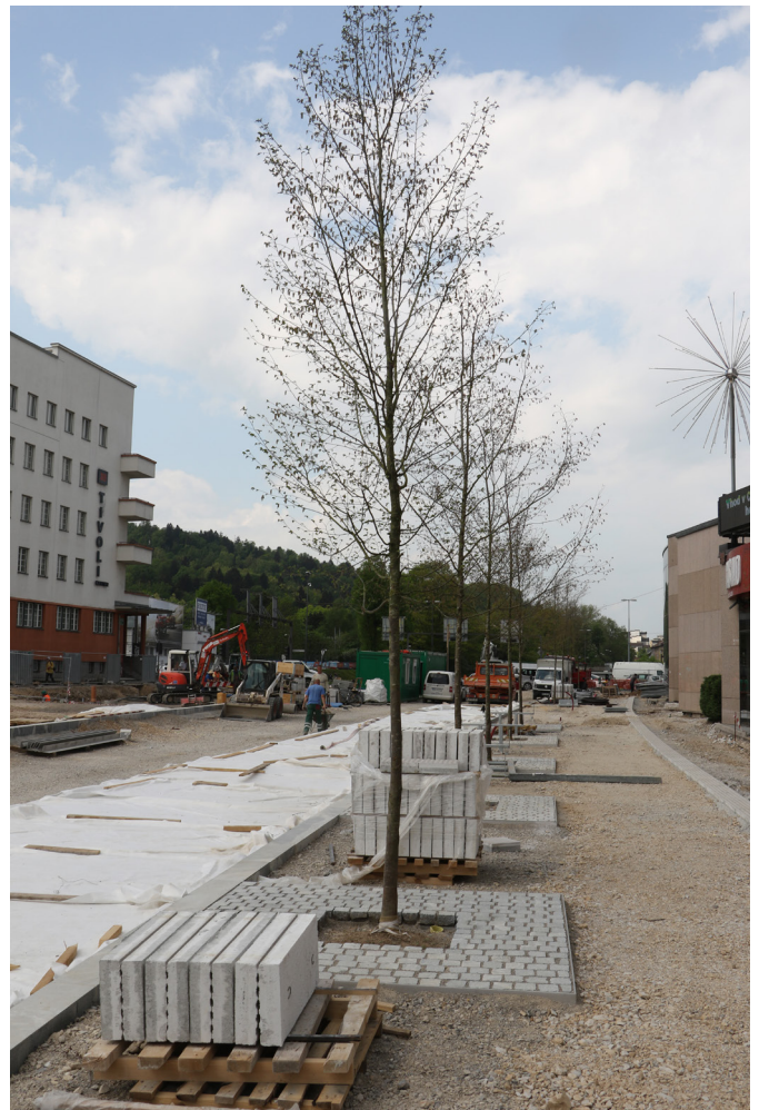
Figure 3: Last renovation of streets in Ljubljana in 2018
