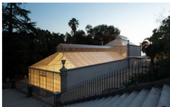
Figure 12: The surrounding area of the greenhouse was also rehabilitated
