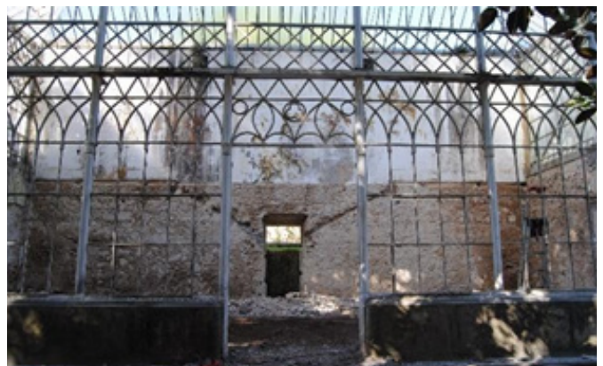
Figure 2: Restoration and rehabilitation
