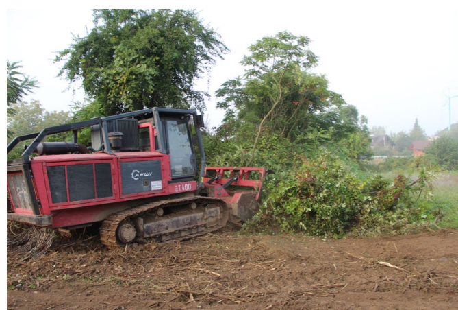
Figure 1: Cleaning the area with a mulcher
