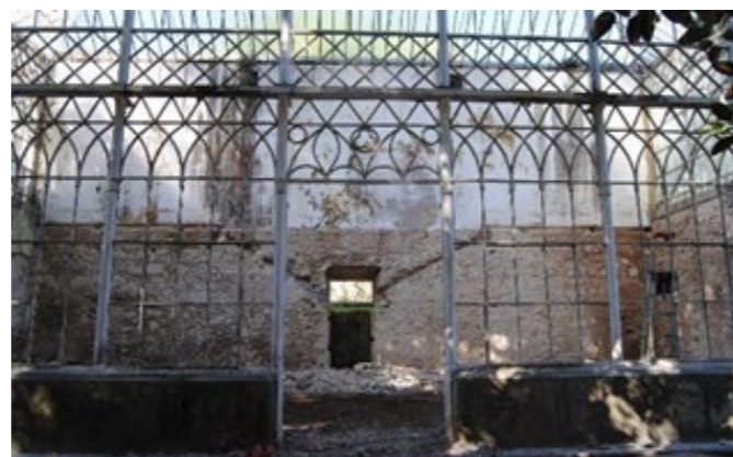
Figure 2: Restoration and rehabilitation
