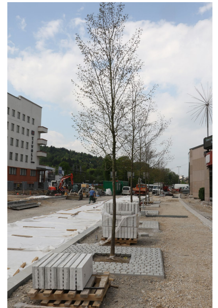
Figure 3: Last renovation of streets in Ljubljana in 2018
