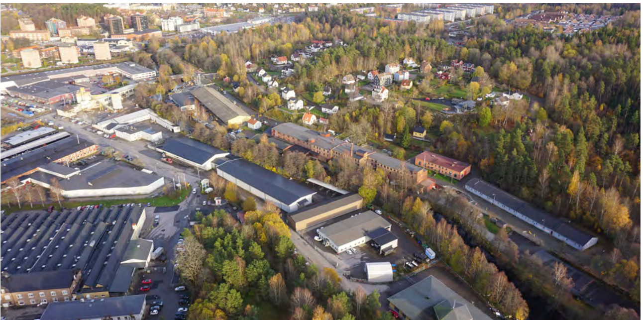
Aerial view of the project site
