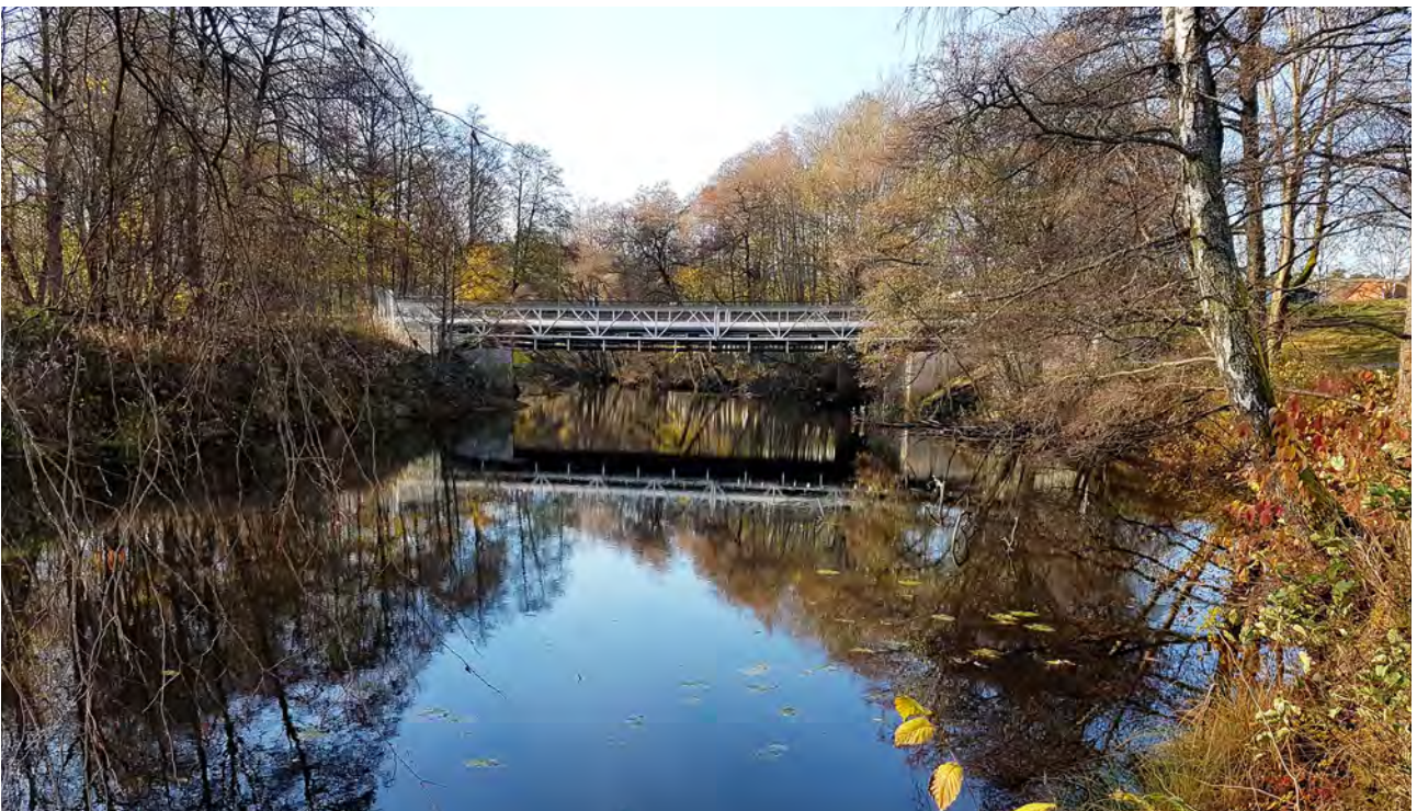
Conduit over Viskan between Gässlösa and Göta
