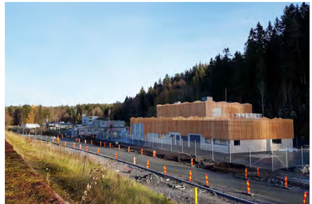
Gässtösavägen and newly built pumping station at the old treatment plant
