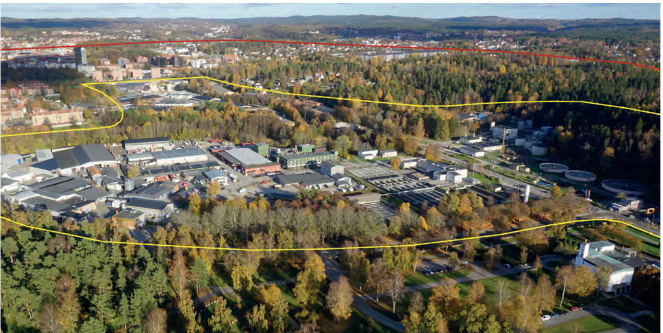
Aerial view of the project site
