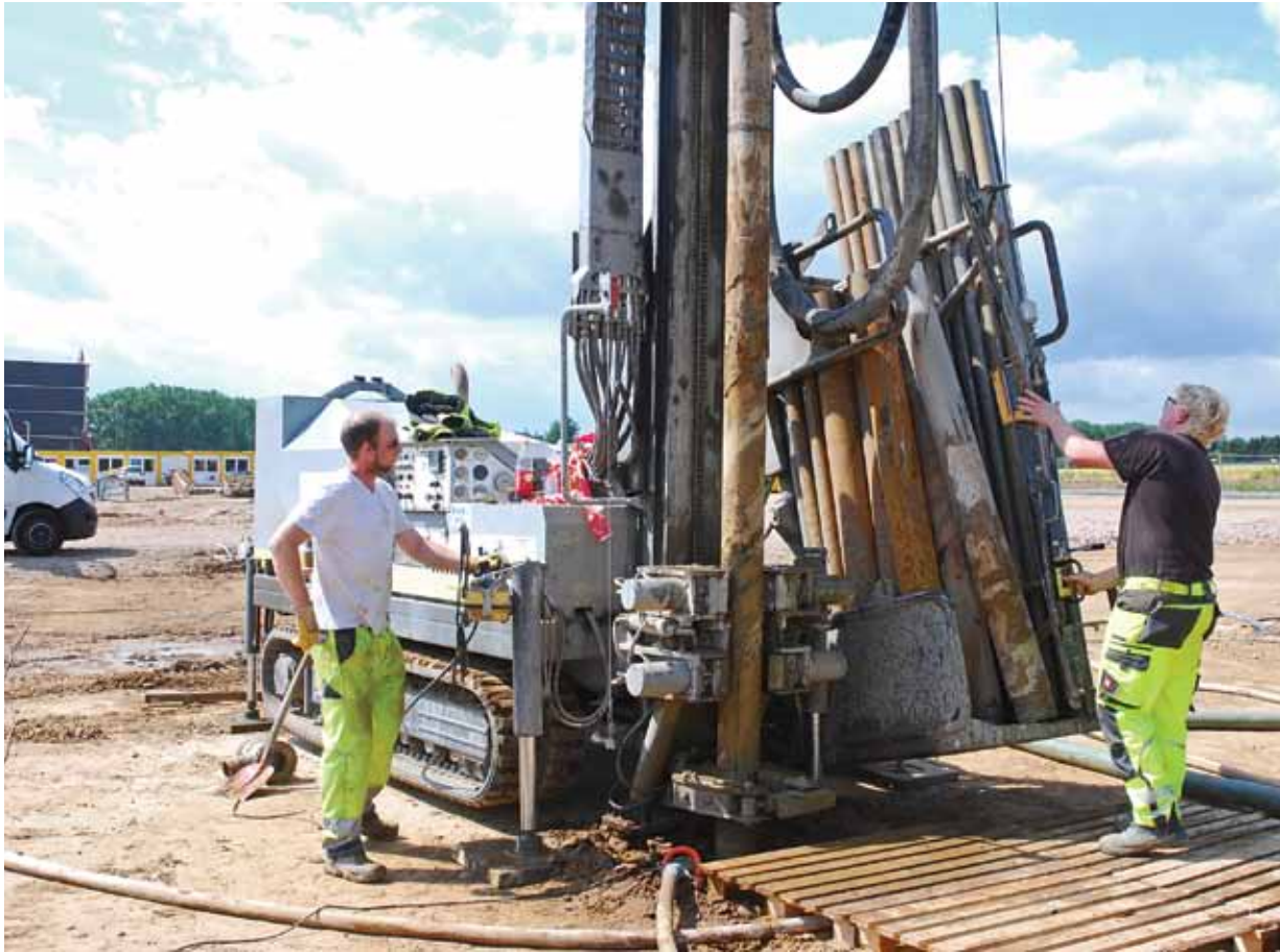
Drilling for Geothermal Energy in TERRA.vita Geopark.
