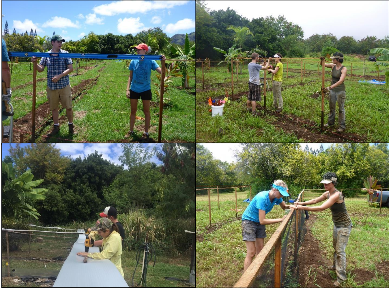
Figure 5. Clockwise from top left, with people identified left to right. Bob Thomson and Robyn Screen checking whether the heights of the upright posts are level. Anthony Barley, Rachel Goodman, and Laci Gerhart-Barley attaching the top frame (the bottom of third of the posts are darkened by copper paint). Robyn Screen and Laci Gerhart-Barley stapling mesh to the frame. You can see the berm of dirt that will be used to refill the trench. Stevie Kennedy-Gold and Marlin Dart attaching the top plastic (Solexx, note how it is one continuous sheet).
