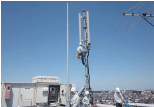
Installation of a base station for mobile phones
