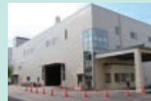
Higashimurayama Recycling Center
