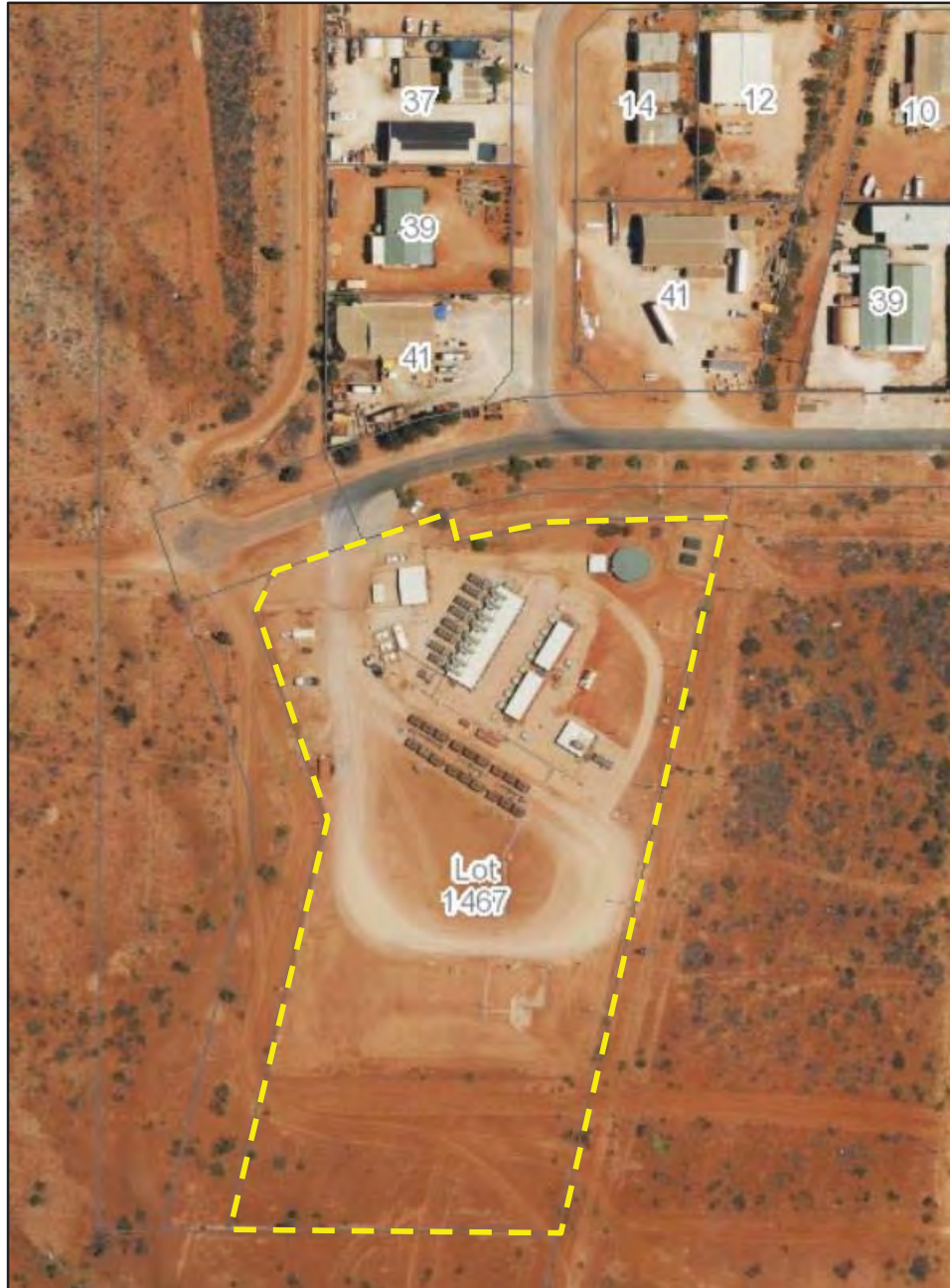
Figure 1: Existing Exmouth Power Station
