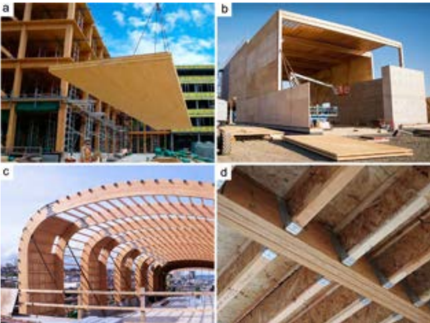
Fig. 13.4 Examples of structural wood-based composites in building construction, (a) CLT and floor panels, (b) MPP roof and wall panels, (c) curved glulam beams with plywood sheathing, and (d) LVL beam supporting composite I-joist and OSB floor sheathing [7].
