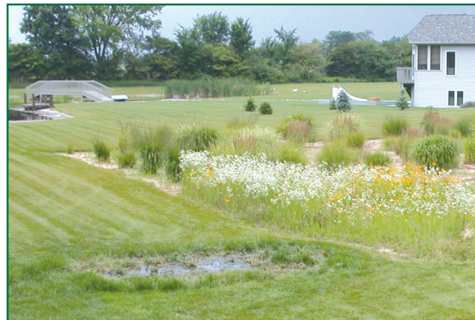
Figure 5. This image shows an example of a failing septic system. Effluent can be seen surfacing on top of the lawn at left.
