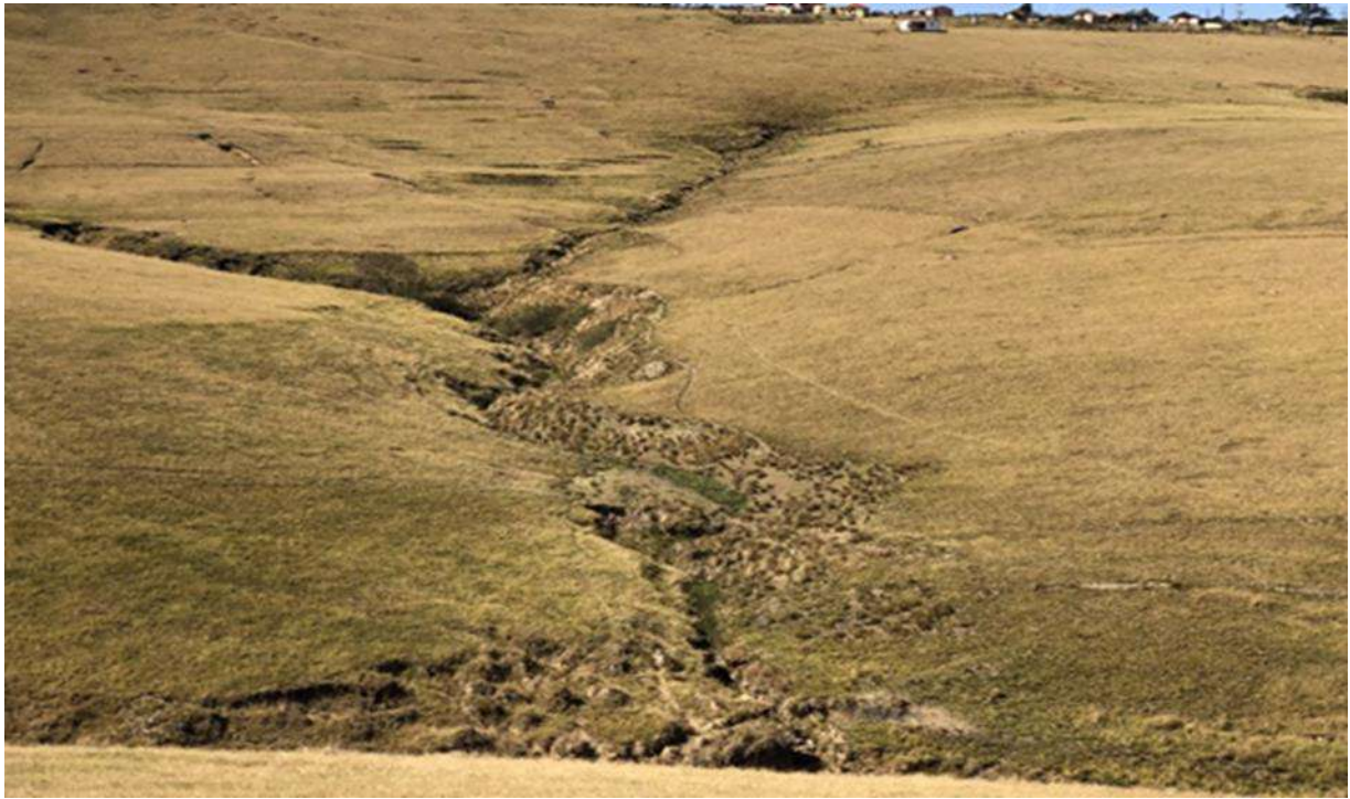
Figure 1: Ridge on the site footprint.
