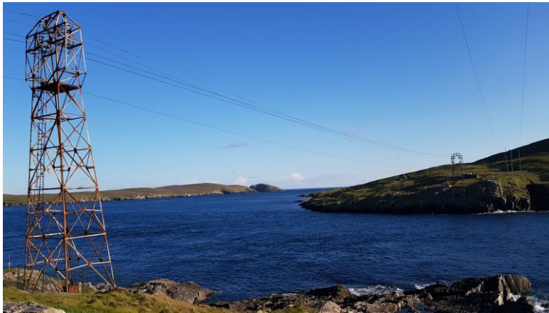
Plate 3.5 View of Dursey Sound and the cable car to Dursey Island.
