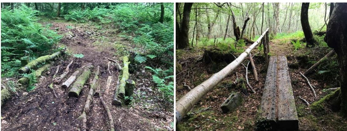
Figure 75 Infrastructure not fit for purpose on the Suck Valley Way
