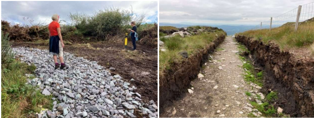
Figure 45 Path built from loose aggregate and cut through deep peat
