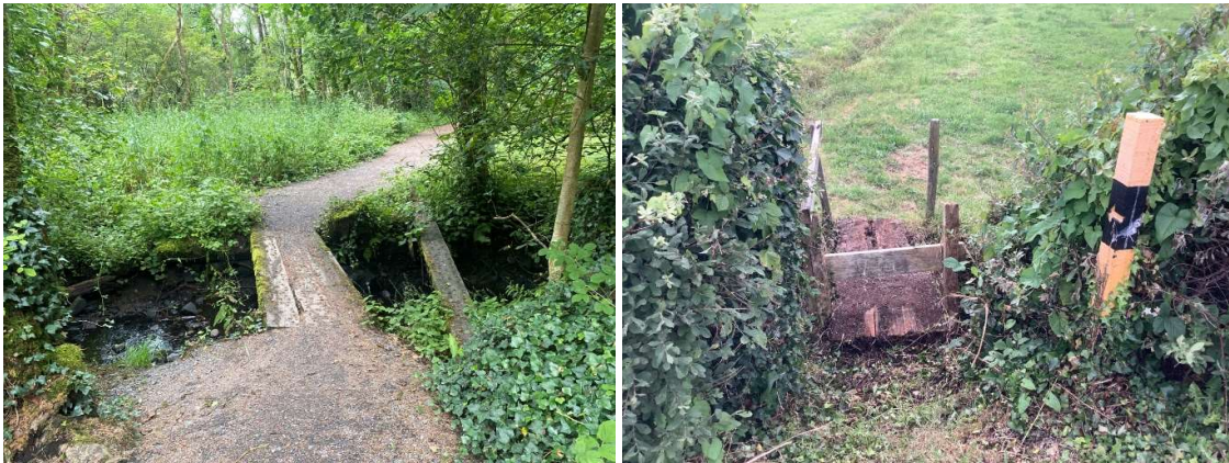
Figure 83 Poor infrastructure on the Miners Way
