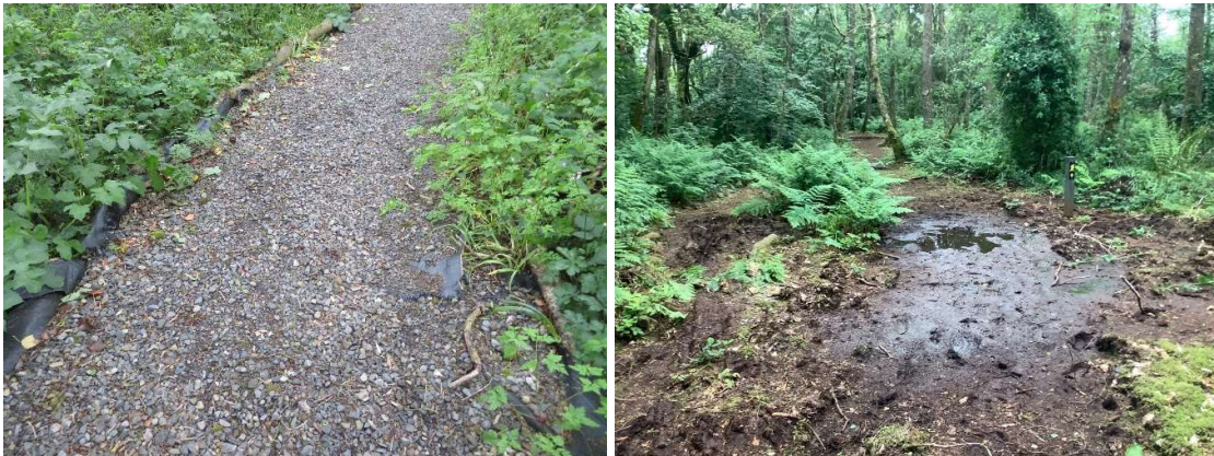
Figure 74 Trail in poor condition on the Suck Valley Way
