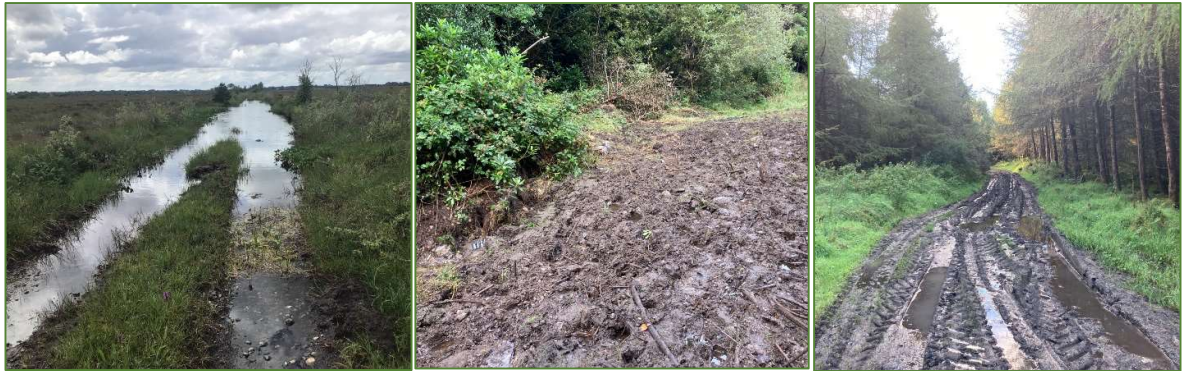
Figure 53 Poor condition trail - standing water, badly poached, damaged by vehicles
