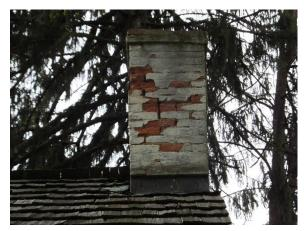
Figure 288. Typical deteriorated condition of the chimney.
