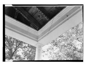
Figure 24. Detailing of the southwest corner of the portico cornice (note ceiling removed during restoration) ca. 1960. (Photo courtesy of HABS).
