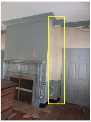
Figure 169. North bumpout at fireplace not reflected on HABS drawings.
