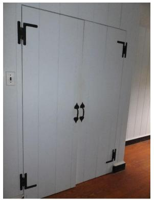
Figure 226. Board and batten closet doors in rooms 205A and B.
