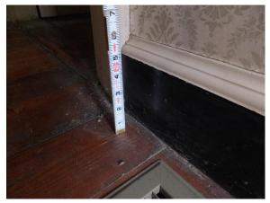
Figure 180. Baseboard height and profiling in room 104 differs than reflected in HABS drawings.
