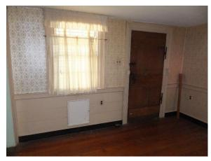
Figure 173. View of east wall of wallpaper, chair rail, and shiplap.
