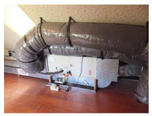
Figure 240. Mechanical unit located at the south wall. Ductwork penetrates through the flooring and walls.
