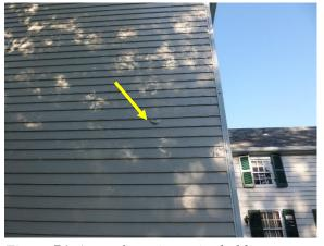
Figure 74. Area of sagging paint holding water on the east facade.
