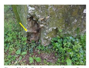
Figure 284. Spall in the concrete "buttress" at the northwest corner.
