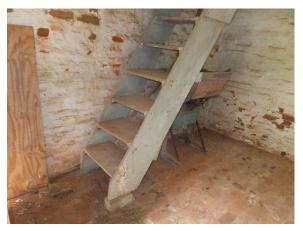
Figure 319. Ladder stairs leading to the second floor.
