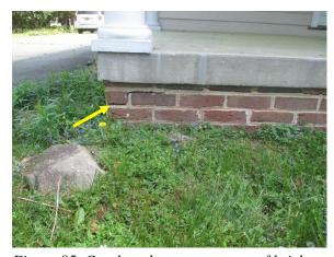
Figure 85. Crack at the upper course of brick at the west patio.
