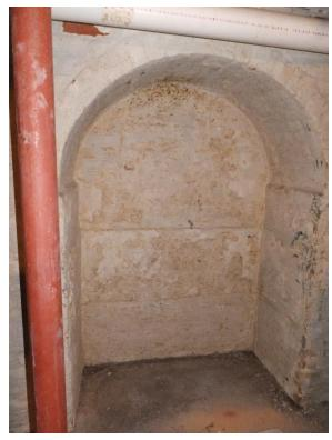
Figure 117. Arched brick masonry support for the east fireplace.
