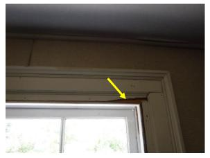
Figure 271. Cracked window trim.
