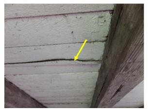
Figure 334. Splintered wood at the underside of the second floor.
