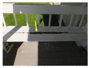
Figure 78. Deteriorated and missing wood at the west bench of the south portico.
