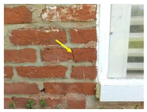
Figure 79. Example of cracking through a brick unit at the brick foundation.
