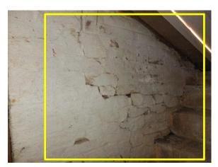
Figure 263. Cracking along the stairs leading to storm hatch.
