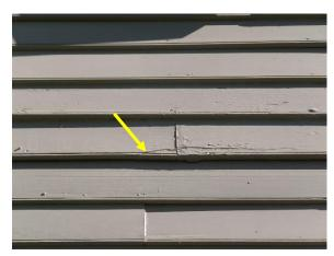
Figure 75. Occurrence of a crack between two pieces of clapboard siding.
