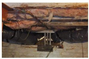
Figure 109. Ventilation window in the basement with view of floor beams and insulation above in 2017.
