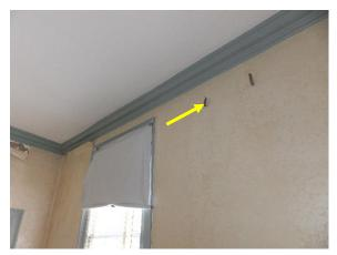
Figure 162. Straps penetrating through the north wall.
