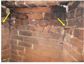
Figure 209. Iron stakes in the firebox embedded in mortar.
