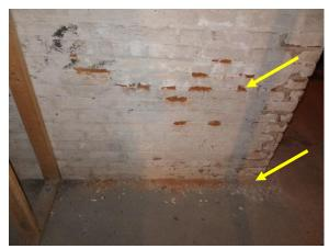
Figure 262. Deterioration of a potentially impermeable coating, likely trapping moisture and contributing to the deterioration of the brick. Note collection of brick debris at the floor.
