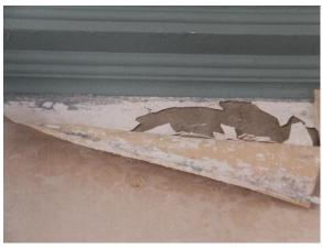
Figure 160. Wallpaper installed on top of white coating applied over sandy plaster.
