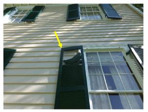
Figure 91. Racked shutter resulting in loose and disconnected slats.
