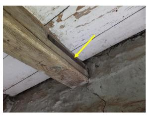
Figure 315. Tie straps tying to star anchor plates at the exterior.
