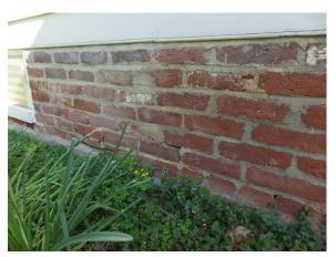
Figure 45. Brick foundation exposed above grade level at the south facade.
