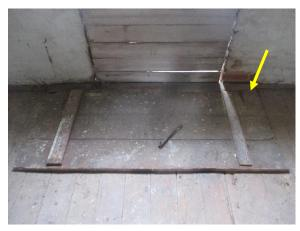
Figure 320. Board and batten hatch between the first and second floors.
