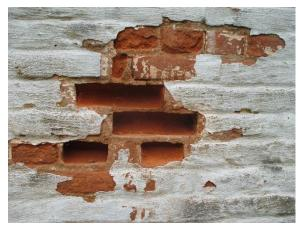
Figure 303. Considerable flaking of impermeable coating with related brick face spalls and deteriorated mortar joints.
