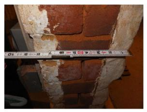
Figure 112. Multi wythe brick wall in the basement with two layers of white coating.
