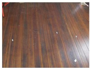
Figure 155. Wood floors in room 103 with signs of smoke contact.
