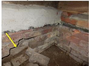
Figure 266. Spalled brick at the foundation under room 102's closet.
