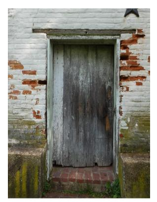
Figure 293. Board and batten door at the south facade.
