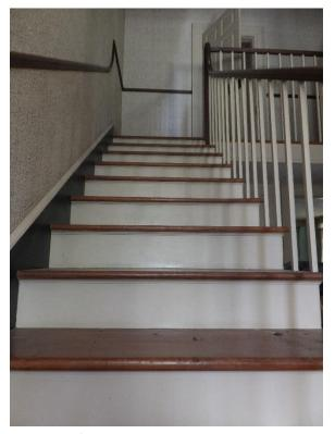
Figure 136. Wood treads with painted risers lead up to intermediate landings.
