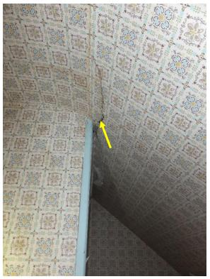
Figure 255. Typical cracking at sloped ceiling to chimney interfaces.
