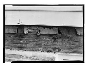
Figure 28. Detailing of wood timber sill on top of the brick foundation exposed during the restoration work ca. 1960. (Photo courtesy of HABS).
