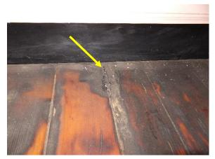
Figure 273. Significant charring of wood floor in room 203.
