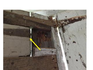
Figure 297. Ghosting of previous straps at batten that has been cut short.
