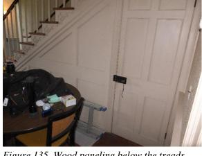
Figure 135. Wood paneling below the treads and ornamentation tying into the paneling of the basement door.
