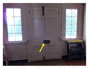
Figure 59. Historic Carpenter's lock with barrel key still in place.
