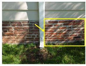
Figure 82. Area of rebuilt brick at the east wing, south facade. Note difference in brick finish and color.
