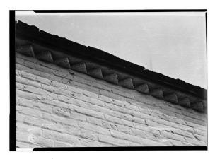
Figure 276. View of dog-toothed brick cornice ca. 1960. (Photo courtesy of LOC)
