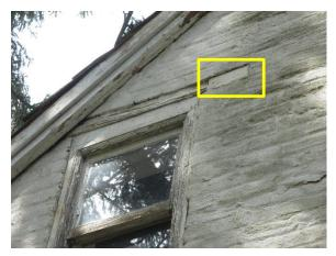
Figure 308. Partial wood dutchman at the east facade window lintel.
