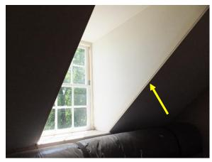
Figure 235. Dormer located at the south wall with wood trim. Note mechanical duct.
