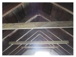
Figure 325. Machine cut roofing members.
