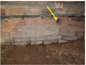
Figure 265. Loose and sagging brick at the foundation under room 102's closet.
