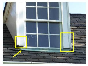
Figure 92. Dutchman repairs were observed at the jambs of dormer windows. Also, note minimal integration of copper flashing at the sill.
