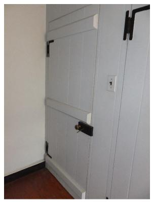
Figure 227. Board and batten doors to rooms 205A and B with horizontal rim locks. Door to 205A still has barrel key in place.
