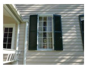
Figure 53. Typical 6/6 wood window with shutters.
