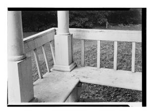
Figure 22. Detailing of the southwest corner of the portico wood benches ca. 1960. (Photo courtesy of HABS).
