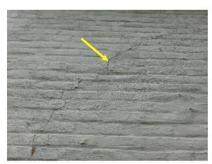
Figure 301. Crack in south facade emanating through the impermeable coating.
