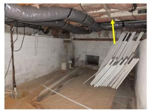
Figure 121. Overview of basement below central section of the home with mostly replaced machine cut floor beams. Note CMU bump-outs and fireplace support.
