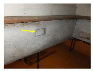
Figure 119. Visible notching of floor beams in the stairwell leading to the basement. Note white coating visible on all structural wood members.
