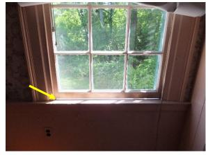
Figure 88. Window at the south facade second floor with 1-inch gap between lower sash and sill.
