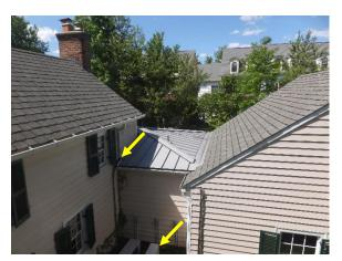
Figure 52. Roof interfaces between central section (left), kitchen/bathroom (center), and garage (right). Downspout from central section gutter deposits water directly onto patio roof. Note mechanical units below.
