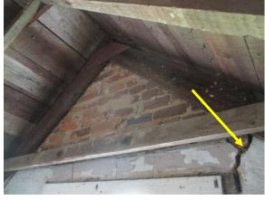
Figure 329. Cracking at the west wall.
