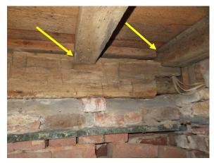
Figure 151. View of floor beams notched to a timber sill looking west.
