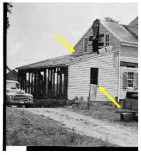
Figure 41. Cropped HABS photograph to show the previous kitchen structure at the north. Note the roof slope and window at the west facade.
