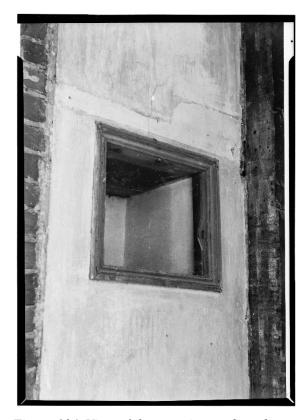
Figure 104. View of the warming cupboard at the south side of the fireplace in room 102 ca. 1960. (Photo courtesy of HABS).
