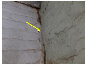
Figure 326. Vertical cracking at wall to chimney interface.
