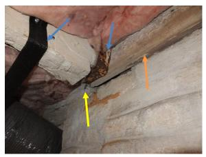
Figure 120. Original timber sill (yellow arrow) cut short and retrofitted with machine cut sill (orange). Note retrofit strap at the floor beam and strap to mechanical duct (blue).
