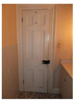
Figure 187. Bathroom door with horizontal rim lock.
