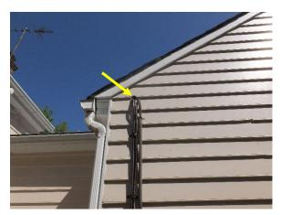
Figure 77. Example of unsealed penetrations through wall cladding.
