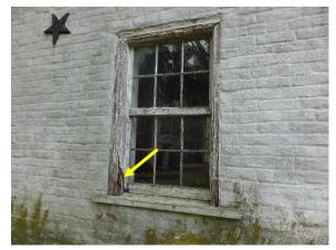
Figure 307. Deteriorated wood with areas of missing material at the jamb.
