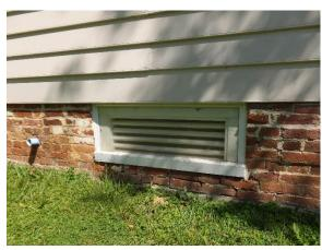
Figure 31. Detailing of wood timber sill on top of the brick foundation with ventilation louver centered in 2017.
