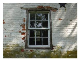
Figure 289. 6/6 wood windows at the first floor on the north and south facades.
