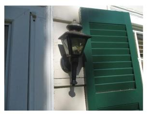
Figure 72. Light fixture added north of the east facade door.
