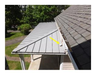
Figure 51. West patio roof interface with central section of the home. Downspout from central section gutter deposits water directly onto patio roof.
