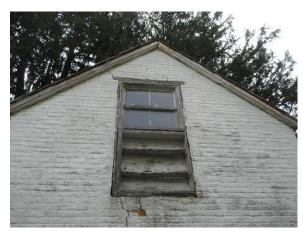
Figure 290. 2/2 wood window at the second floor west facade with wood shelves below.
