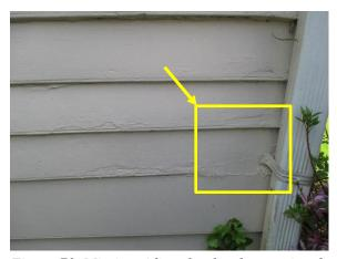
Figure 73. Missing siding that has been painted over, adjacent to a downspout.
