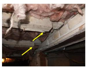
Figure 114. Original floor beams short of original bearing point.
