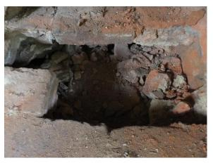
Figure 333. Brick removed to reveal loose gravel below.
