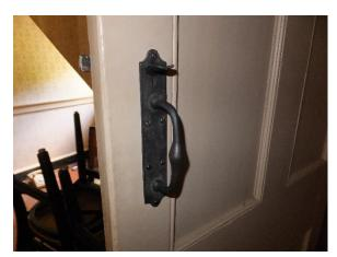
Figure 177. Stair door has a thumb latch and door pull.
