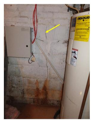
Figure 261. Crack in CMU at central section foundation.
