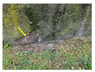
Figure 283. Stone visible in an area of delaminated parge coating.
