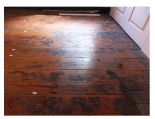
Figure 214. Charring of wood floor in room 203
