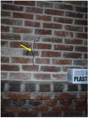
Figure 264. Cracking at fireplace in kitchen. Cracks traced for clarity.
