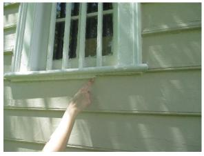
Figure 89. Area of missing trim below sill of east wing window.
