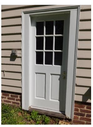
Figure 65. Typical upper divided light exterior doors at the garage.
