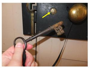
Figure 60. Barrel key for the main door. Note Carpenter & Co. Patentees seal with British Royal Arms centered.
