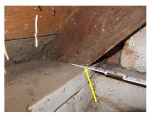
Figure 335. Numerous rafters near the gable ends are not fully bearing on the plate.
