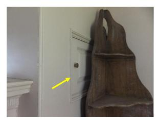
Figure 147. Warming cupboard at the south face of the chimney.
