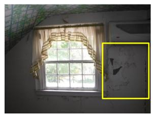
Figure 258. Damage to interior finishes below a mechanical unit.
