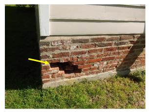
Figure 83. Area of spalled brick at the west wing, south facade.
