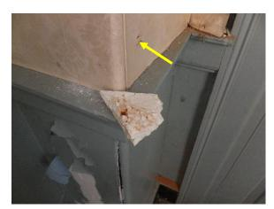
Figure 161. Wall sheathing applied around fireplace evidenced by screws.
