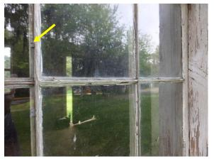
Figure 306. Complete loss of glazing putty with glazing points exposed at the north window.
