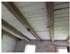
Figure 314. Hand hewn floor beams running north to south.
