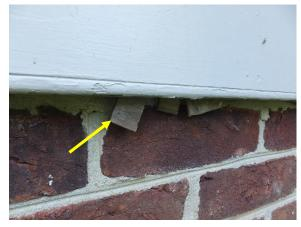
Figure 76. Shims observed between the clapboard siding and brick at the garage.
