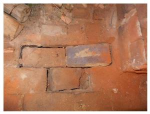
Figure 332. Loose brick in the floor adjacent to firebox.
