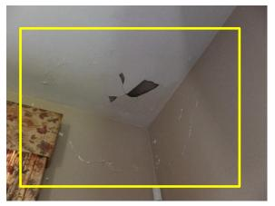
Figure 249. Typical plaster damage at the first floor.
