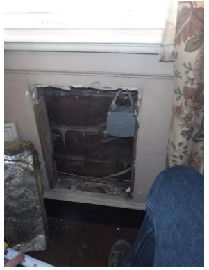
Figure 152. Access hatch removed in room 102 revealing backside of clapboard siding.
