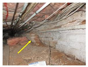
Figure 126. Partially demolished wythe of brick at the east wall.
