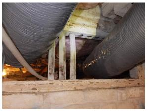
Figure 116. Original ventilation openings that are utilized for mechanical ductwork pathways.
