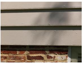
Figure 29. Wood clapboard siding currently obscures the wood members in 2017.
