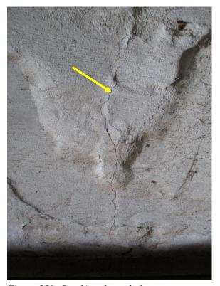
Figure 330. Cracking through the parge coat.
