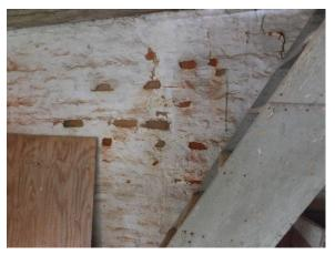
Figure 328. Flaked coating with cracked and spalled brick at the west wall.
