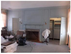
Figure 210. Fully paneled east wall with contemporary bathroom (left) and closet (right) paneled doors.
