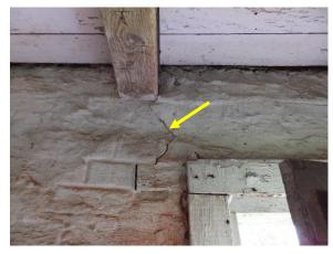
Figure 327. Cracking emanating from floor beam connection.
