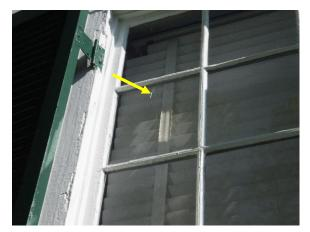
Figure 87. Example of cracked glazing lite.
