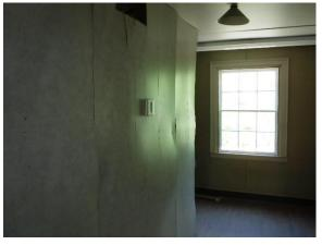
Figure 260. Warped wall paneling in the garage upper space.
