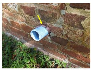
Figure 84. Flexible hose penetration through the brick foundation at the south facade.
