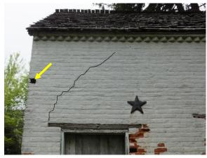
Figure 285. Missing brick at southwest corner. Note adjacent crack to the right emanating from door lintel. Cracked traced for clarity.
