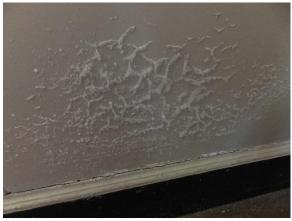
Figure 251. Gypsum salt crystallization of plaster.
