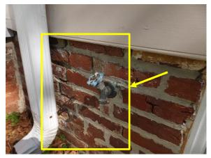
Figure 81. Areas of missing mortar adjacent to a downspout and spigot.
