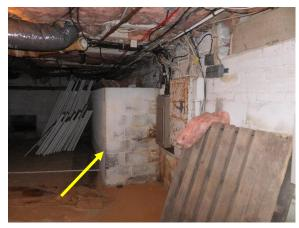
Figure 125. Partial CMU foundation and bumpout at the east wall below the central section of the home.
