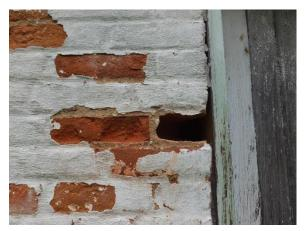
Figure 302. Flaked impermeable coating with related brick face spalls and missing brick.
