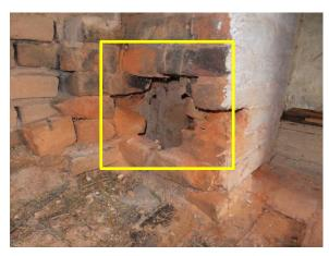
Figure 331. Spalled area of brick in the second floor firebox.
