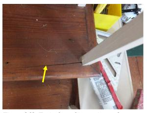
Figure 268. Typical cracking stair treads.
