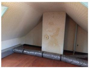
Figure 257. Typical water staining at the wallpaper at the third floor.
