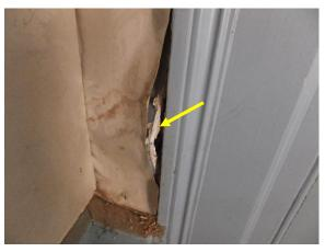
Figure 158. Damaged wall finish, gypsum board, adjacent to false door.
