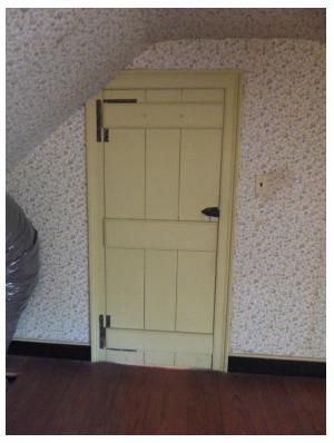
Figure 237. Interior board and batten door to room 302.
