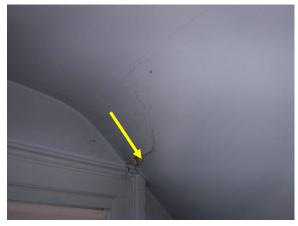
Figure 254. Typical cracking at sloped ceiling to wall interfaces.
