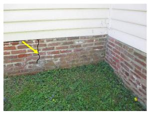
Figure 80. Crack through numerous brick units on the west facade. Crack traced for clarity.
