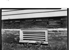
Figure 30. Detailing of wood timber sill on top of the brick foundation with ventilation louver centered ca. 1960. (Photo courtesy of HABS),
