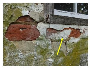
Figure 279. Flaked impermeable coating reveals what appears to be a lime wash.
