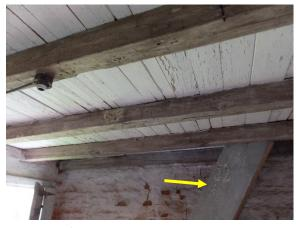
Figure 316. Ladder stairs nestled between floor beams at the west wall.
