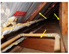
Figure 242. View into the access hatch looking east reveals machine cut rafters, stud framing, and joists.
