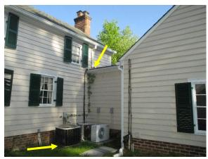
Figure 94. East facade with downspout of central area emptying water on bathroom roof and onto mechanical units. Note vegetation growth in this area.
