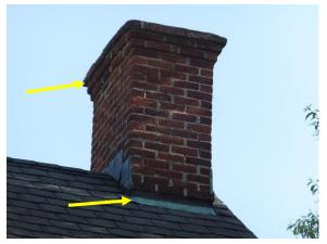
Figure 95. Chimney with no cap flashing and minimal integration of step flashing at roofing assembly.
