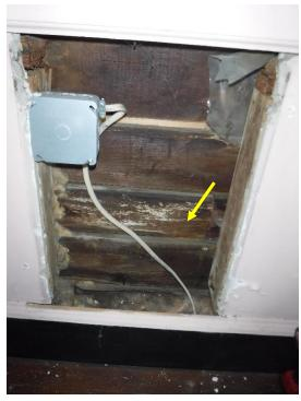
Figure 221. Access hatch opened in room 203 revealing backside of clapboard. Note white coating on one board.
