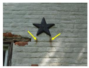
Figure 305. Corrosion staining from the iron star plate.
