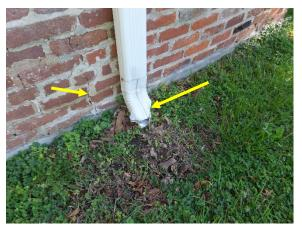
Figure 93. Typical downspout without splash pad or extension. Note adjacent crack through brick units (left of downspout).
