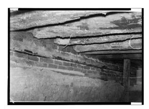
Figure 110. Floor beams in the basement bearing on the brick masonry foundation ca. 1960. (Photo courtesy of HABS).
