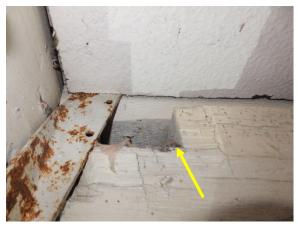
Figure 124. Original timber sill at the west wall with a bearing pocket cut for the floor beams
