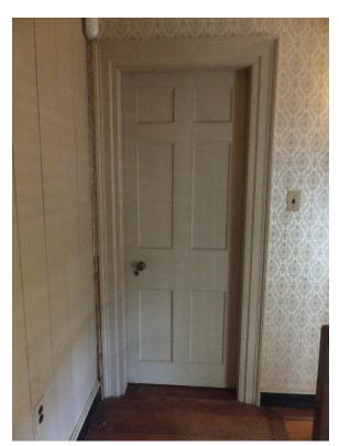
Figure 222. Door leading from room 204 to the intermediate landing of grand stairs. Doorway to stairwell was originally located to the west (right) and aligned with stairs.
