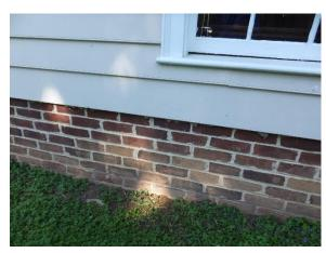
Figure 46. Exposed brick at the garage addition with grapevine tooled mortar.
