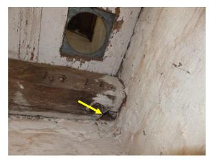
Figure 317. Triangular cut in beam #8 at west wall.
