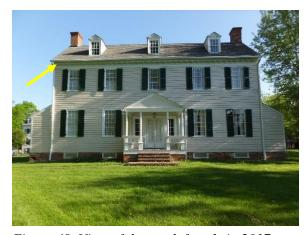
Figure 49. View of the south facade in 2017 revealing 37 modillions with 8 dentils between each modillion along the cornice.
