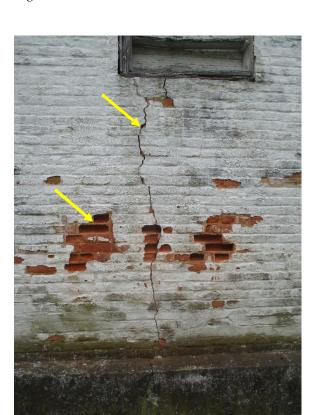
Figure 300. Significant vertical crack, flaked coating, and brick face spalls at the west facade.
