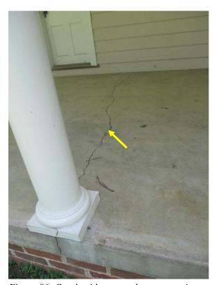
Figure 86. Crack midspan on the west portico.
