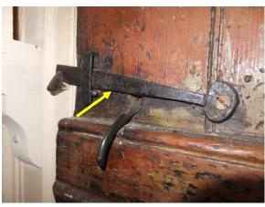
Figure 64. Wrought iron latch at the interior of the board and batten door.
