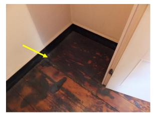
Figure 215. Significantly charred northwest corner of the closet.
