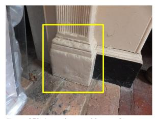
Figure 270. Area of material loss at chimney that has been painted over.
