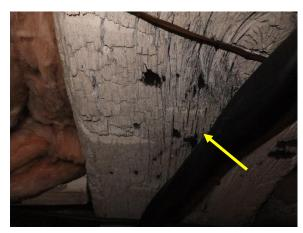
Figure 123. One original rough hewn floor beam remaining below the central section that is charred with a white coating.
