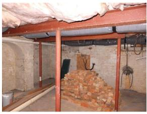
Figure 113. View into the east room of the basement showing poured concrete floors with retrofitted steel beams and lally columns. Brick in photo is from the floor of the meat house.
