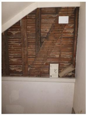
Figure 103. View of the only visible plaster and lathe wall below grand staircase looking west in 2017. Not the same location as the HABS photo.
