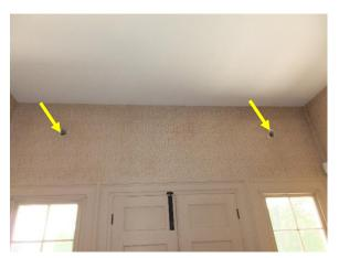
Figure 247. Holes in wallpaper and plaster ceiling above the main entry doors.
