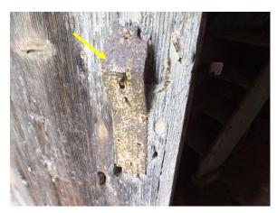
Figure 294. Wrought iron thumb latch.
