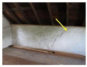
Figure 324. Partial parge coating observed at the second floor.
