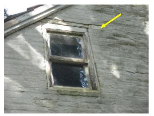
Figure 291. 1/1 wood window at the second floor east facade. Note previous dutchman at lintel.
