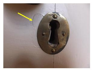
Figure 141. Key escutcheon with evidence of previous hey hole location.
