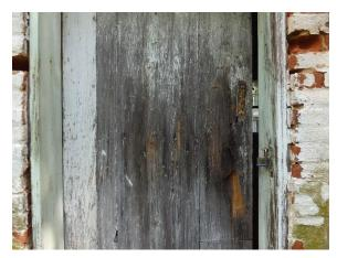
Figure 309. Exposed wood and wrought iron hardware at the board and batten door.
