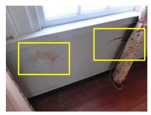
Figure 252. Moisture damage to the east wall of room 105 adjacent to exterior mechanical units.
