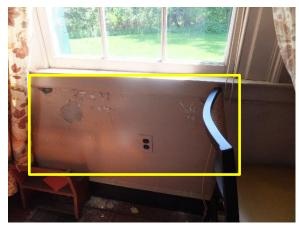
Figure 250. Typical water infiltration damage below windows.
