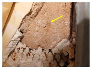
Figure 159. Removal of the damaged wall finish of gypsum board reveals white gypsum material with metal lathe and sandy material with embedded hairs.
