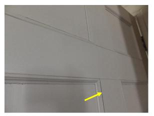
Figure 267. Typical separation of door joinery.
