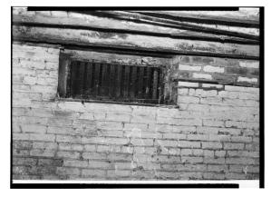
Figure 108. Ventilation window in the basement with view of floor beams above ca. 1960. (Photo courtesy of HABS).
