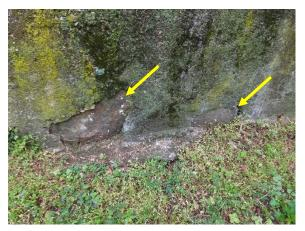
Figure 299. Area of parge coating delamination revealing stone. Note biological staining.
