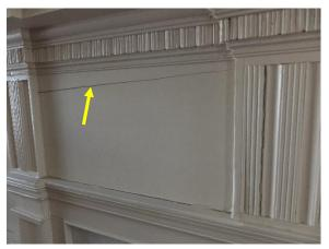
Figure 269. Typical cracking in fireplace ornamentation.
