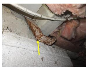
Figure 122. Example of retrofit strap from floor beam to timber sill at the west wall.
