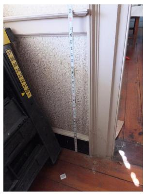
Figure 131. View of typical chair rail and baseboard profiling and orientation throughout the majority of the house.
