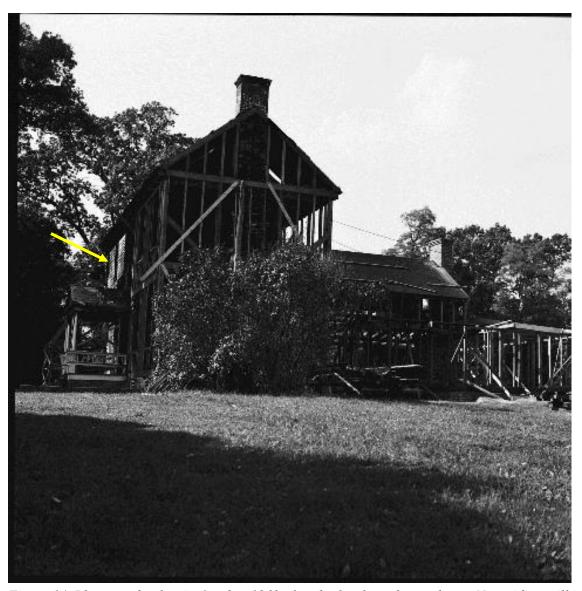
Figure 14. Photograph taken in October 1960 after the fire from the southeast. Note siding still intact along southwest.
