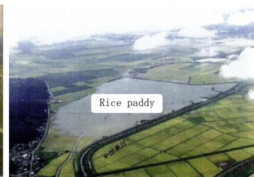
Photo 2-15 Nabirenuma flood control basin (Misato Town, Wakuiya Town)
