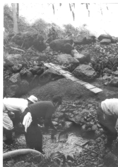
Photo 41 Repair Work Following the Kano River Typhoon
