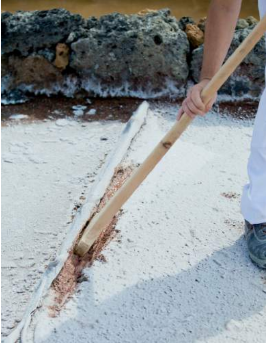
Repair work on the edges of the salt-pans.
