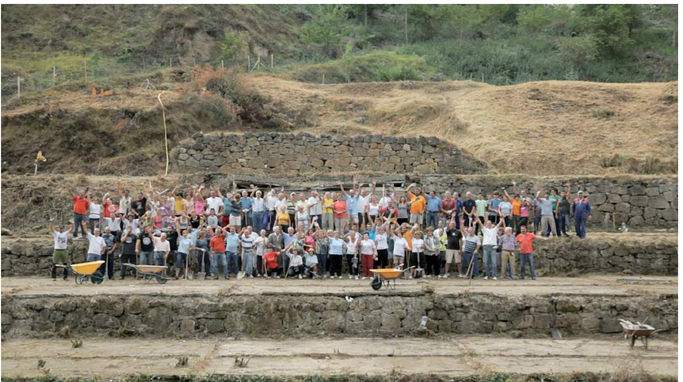
The Local Community performing recovery and maintenance work in the salt cultivation areas.
