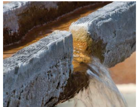
The distribution channel with the opening that allows the brine to fill private wells.
