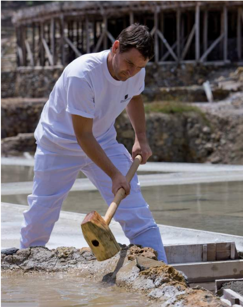
Using a "machuqueta" to waterproof a well with clay.
