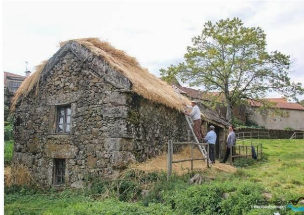
Photo 37. Restored thatched roof of the fulling mill, Paredes do Rio, municipality of Montalegre.
