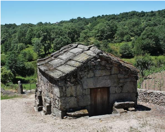
Photo 41. People's oven in Travassos da Chã, municipality of Montalegre.
