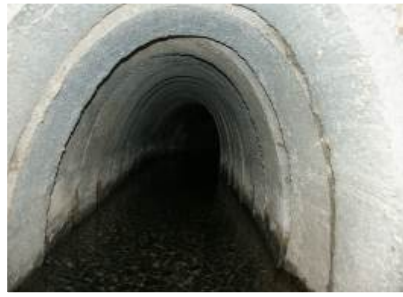
Concrete lining of the qanat gallery
