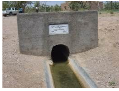
Reconstruction of the qanat outlet
