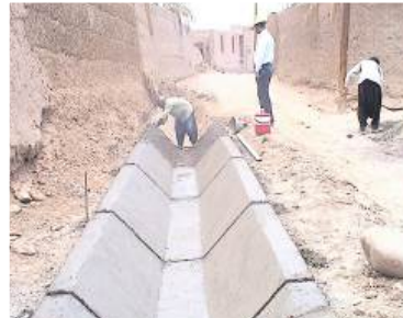
Concrete lining of the open canals
