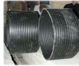
Poly-ethylene pipes for lining the qanat gallery
