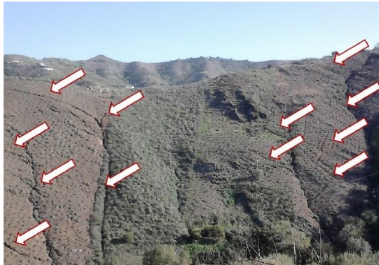
Fig. 32. Water flowing to the drains in a slope of the area. Picture by Jesús Comino
