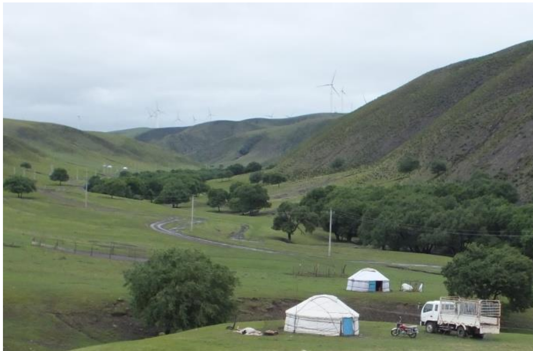
Fig2.2.43 The prospect is the wind electricity field in Talinhua Area
