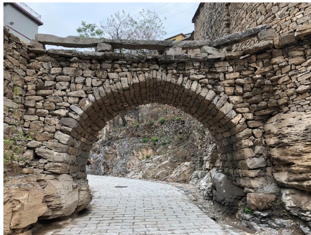
Fig. 2.2.30 Arch Bridge of “Suspended Arch Mosaic” Structure
