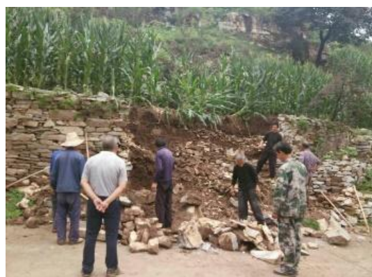
1: Clearing the Area
