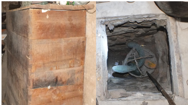
Fig. 2.2.49 Xuan (Left) and Cellar (Right)
