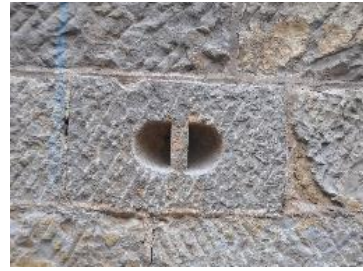
Stone Ring (to temporarily leash livestock)
