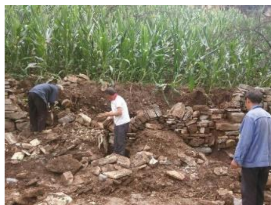
2: Digging to Foundations
