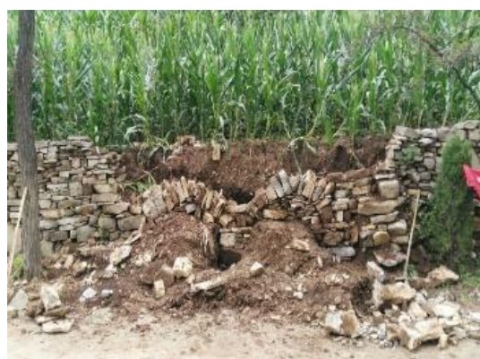
3: Building the Arch
