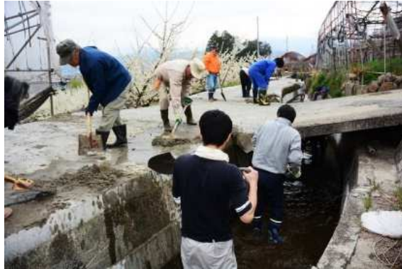
Photo 51. Maintaining segi water channels
