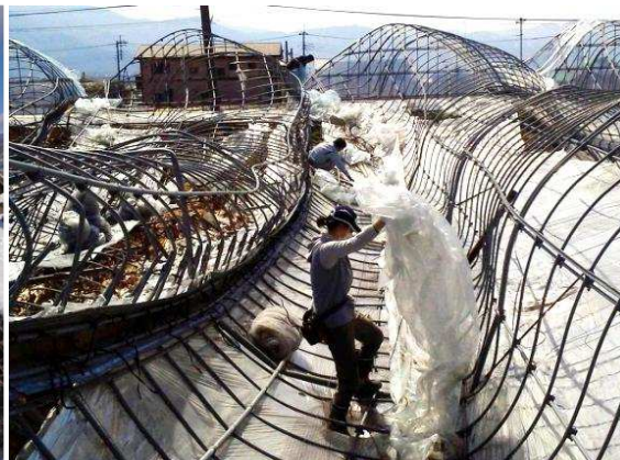
Photo 45. Agricultural facilities damaged by heavy snows in 2014
