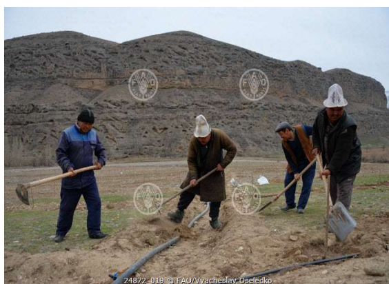
Subsurface drip irrigation with drip tubes buried ©FAO
