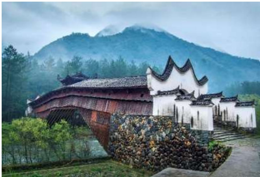
Figure 64 Langqiao (Corridor Bridge) formed by building gallery houses on the bridge deck. Gumin built a large number of Langqiao to facilitate the crossing of the river and to provide shelters for passers-by in the site.
