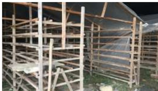
Mushroom shed construction
