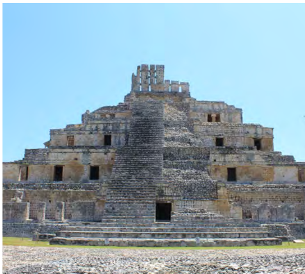
FIVE STORY BUILDING, EDZNÁ, CAMPECHE. PHOTO: GILBERTO M. GONZÁLEZ KUK
