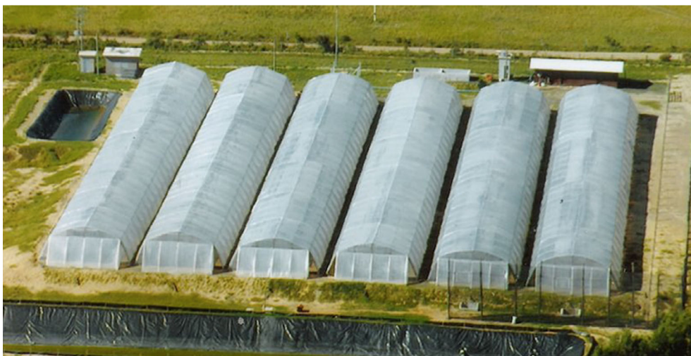
FIGURE 4 Bio-RAS with six greenhouse fattening reactors, recirculation tank (bottom) and denitrifying tank or sludge concentration/reuse tank (top left). Photo: Sergio Zimmermann (2003).
