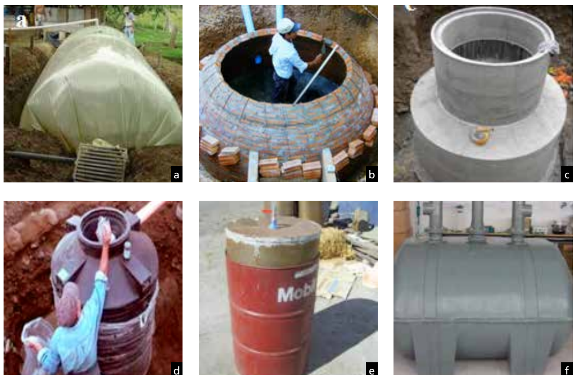
Figure 4 Different materials used for the construction of biodigesters: a) plastic sleeves; b) brick; c) concrete; d) recycled plastic drums; e) recycled metal drums; f) prefabricated
