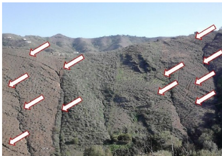
Fig. 32. Water flowing to the drains in a slope of the area.
