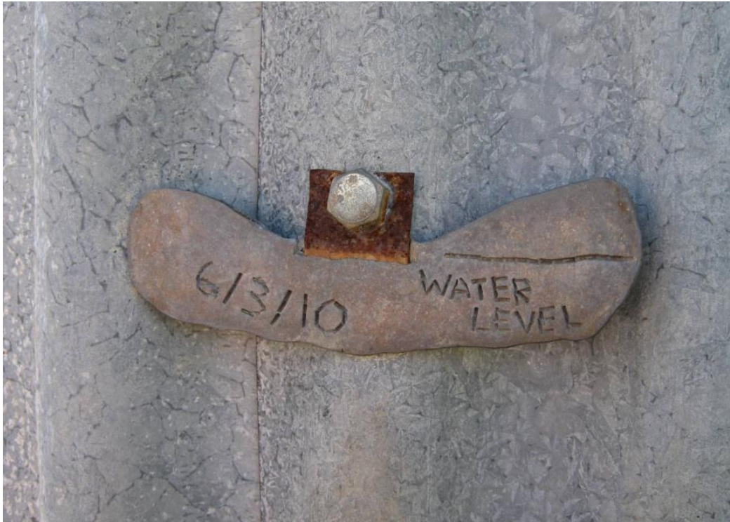
Figure 16. 2010 flood level engraving on the McIntyre's engine shed wall, March 2013
