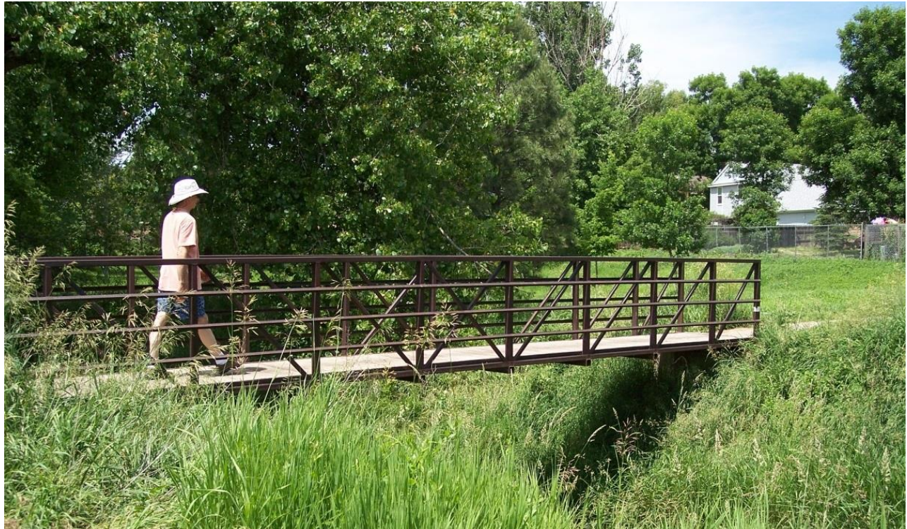
Neighborhood access at Fischer Natural Area
