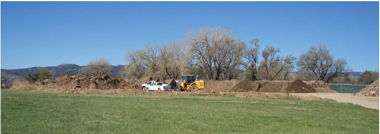
Stormwater Utility storage area at Site #13IS1
