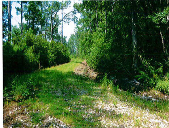
WeSF Figure 2: Some forest roads and associated road ditches interrupt and divert a significant amount of wetland surface flow from their natural drainage patterns on Welaka State Forest.
