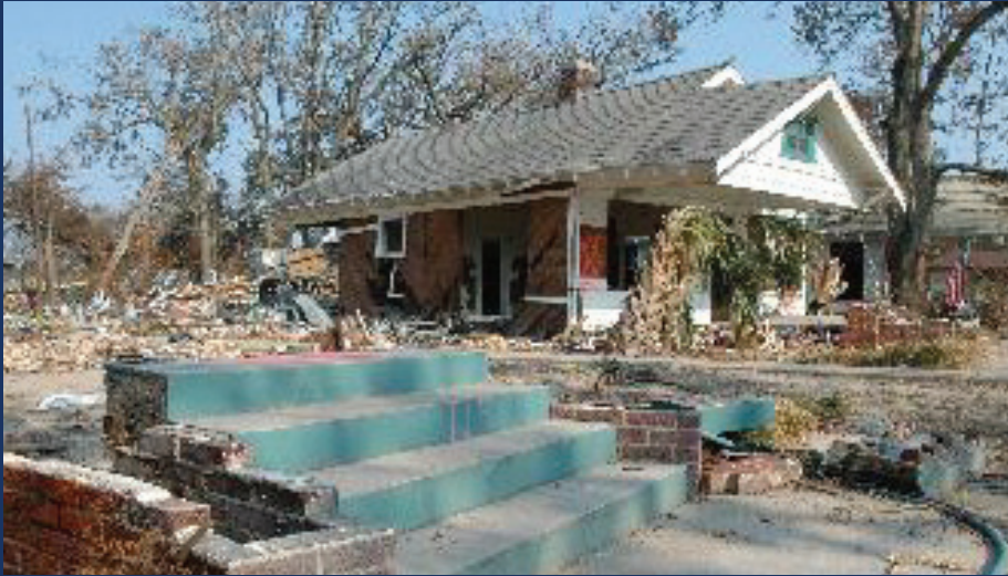
Exhibit 1-2: Damage from Hurricane Katrina.
