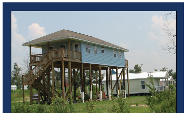
Exhibit 3-2: Elevation requirements vary along the Mississippi Gulf Coast. Elevated home in Waveland, MS; July 2008.
