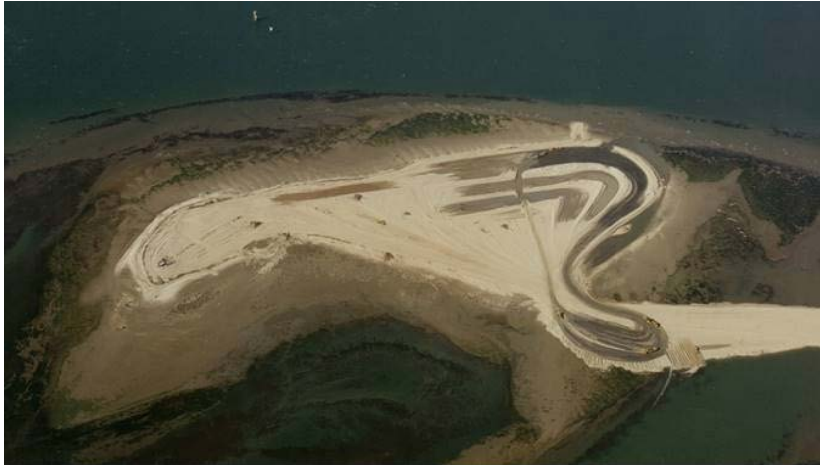
Figure 2-7. Partial removal of the spoil island, used as a source of fill for Runway 4/22 extension (1987), photo by Ward Robertson
