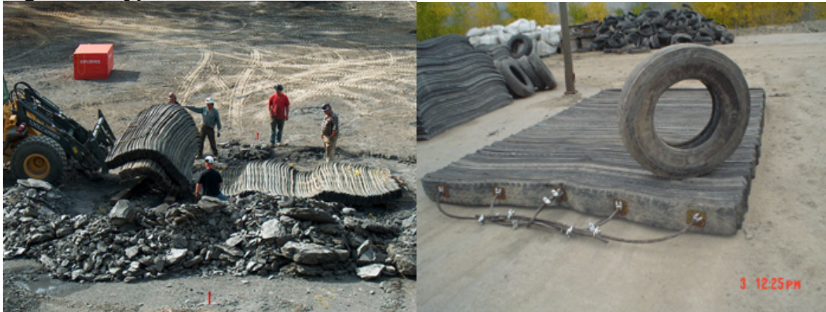
Figure 3. Typical Blast Mats Made from Used Tires
