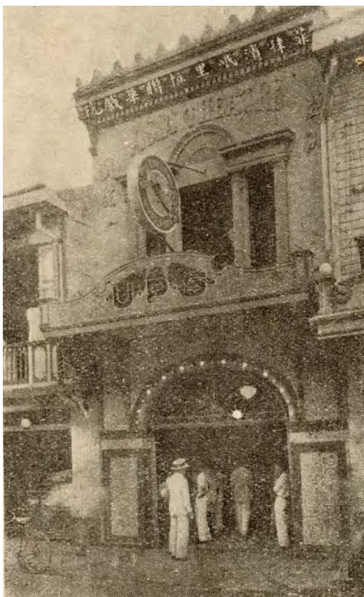
The UPS Theatre in Manila, the Philippines
