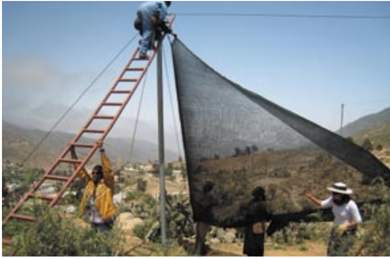
Due to strong winds, installing the fog nets in Nefasit becomes an acrobatic feat.
