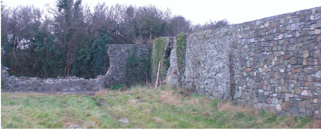
Plate 36 The Garden walls have been partially reconstructed
