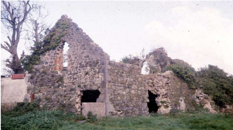
Plate 13 The kitchen extension in 1985 (after Healy) showing a complete gable end with a narrow opening in it with brick repair. There is a pointed Gothic doorway on the first floor of this extension which would have lead to the head of the stairs in the main hall-house structure, for which there was evidence of a stairwell.
