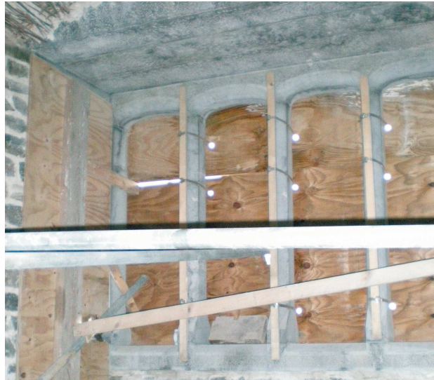
Plate 26 Third Floor view of oriel window in the south gable
