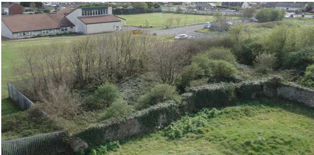
Plate 5 View of the church and graveyard, attached to the southwestern corner of the walled garden, entirely overgrown with dense vegetation
