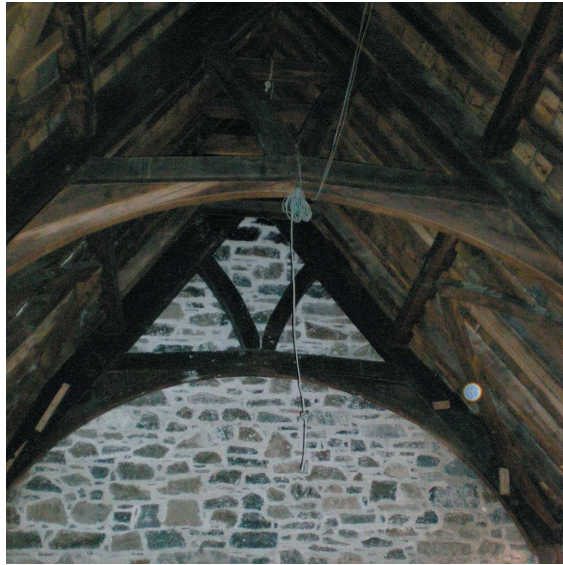
Plate 32 View of reconstructed timber roof to kitchen wing extension
