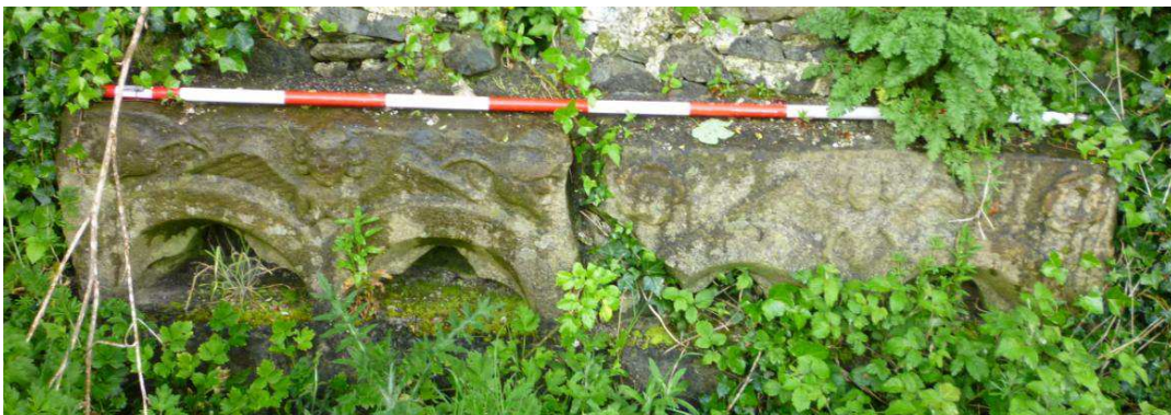
Plate 41 Carved fragment, two ogee headed windows in the graveyard, bonded to the wall
