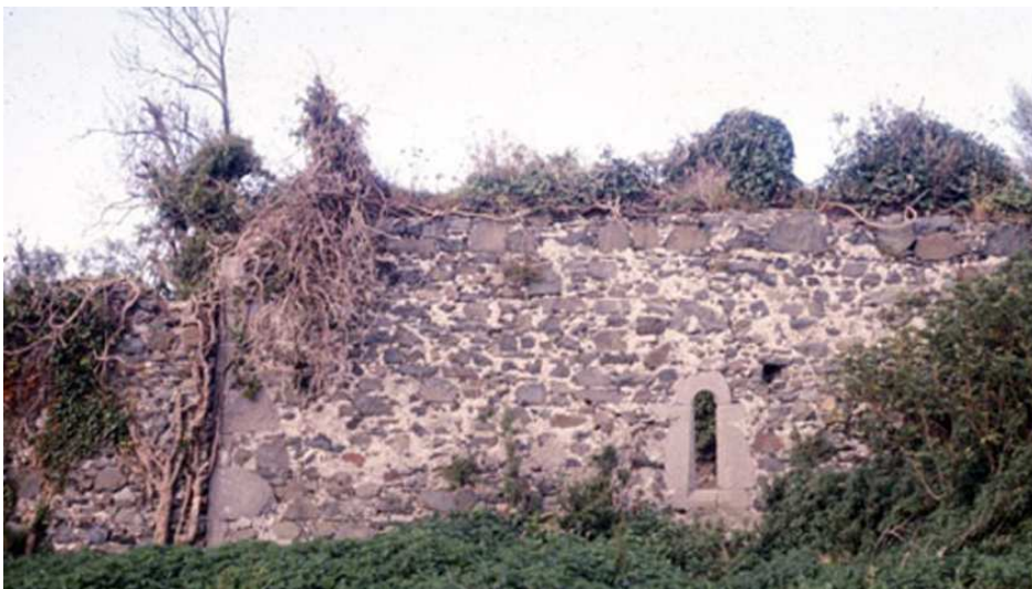
Plate 14 The south-western wall of the hall-house, centrally placed is a round headed loop with a tapering external chamfer and inward splay, this is typical sixteenth century type (after Healy 1985)
