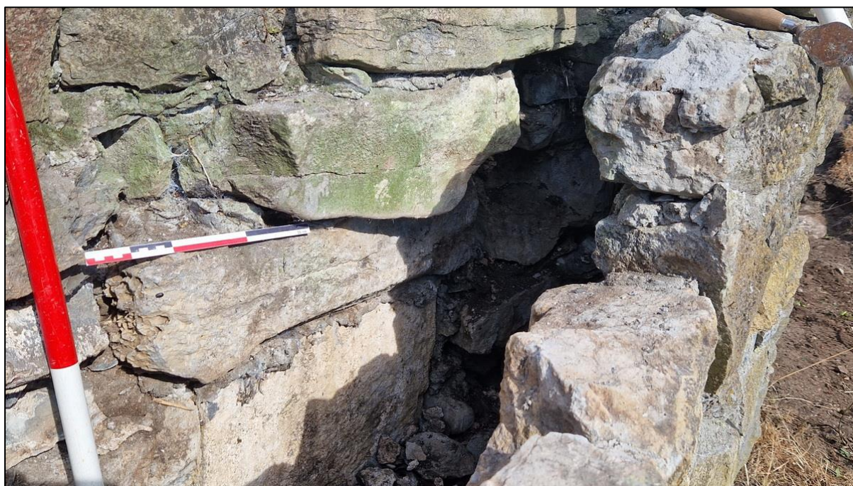
Plate 14 Cill rebuilt into south wall (below small scale), with larger stone directly below
