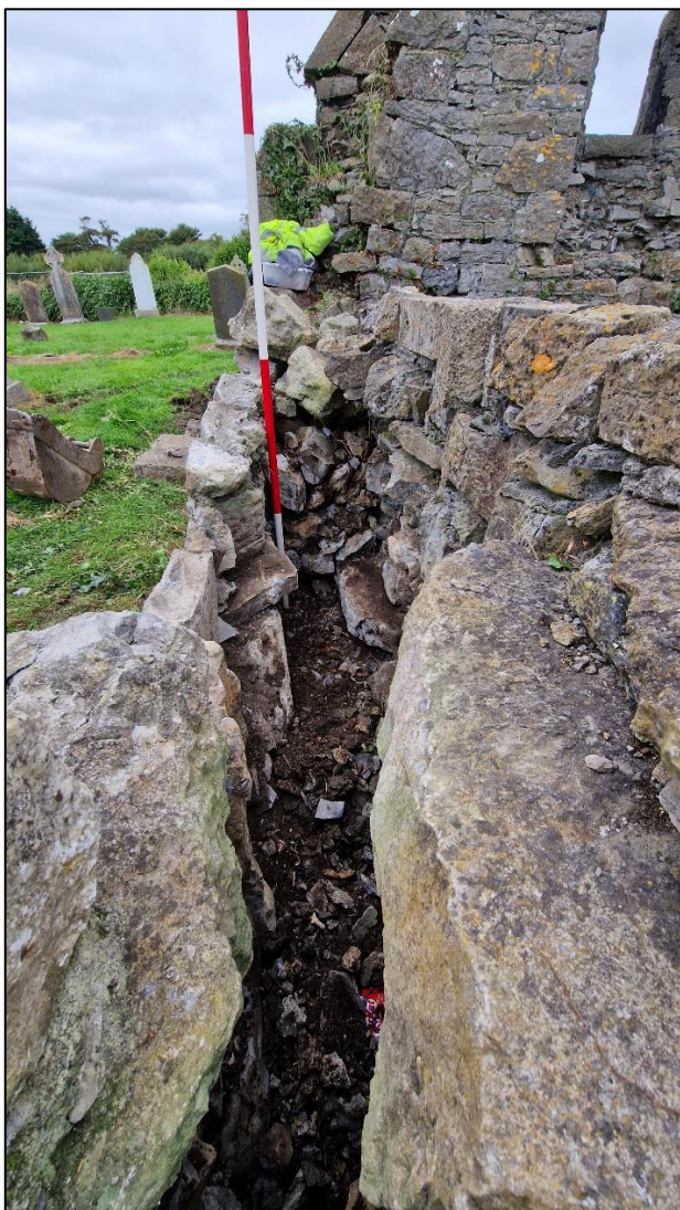
Plate 13 Void within south wall, west of entrance
