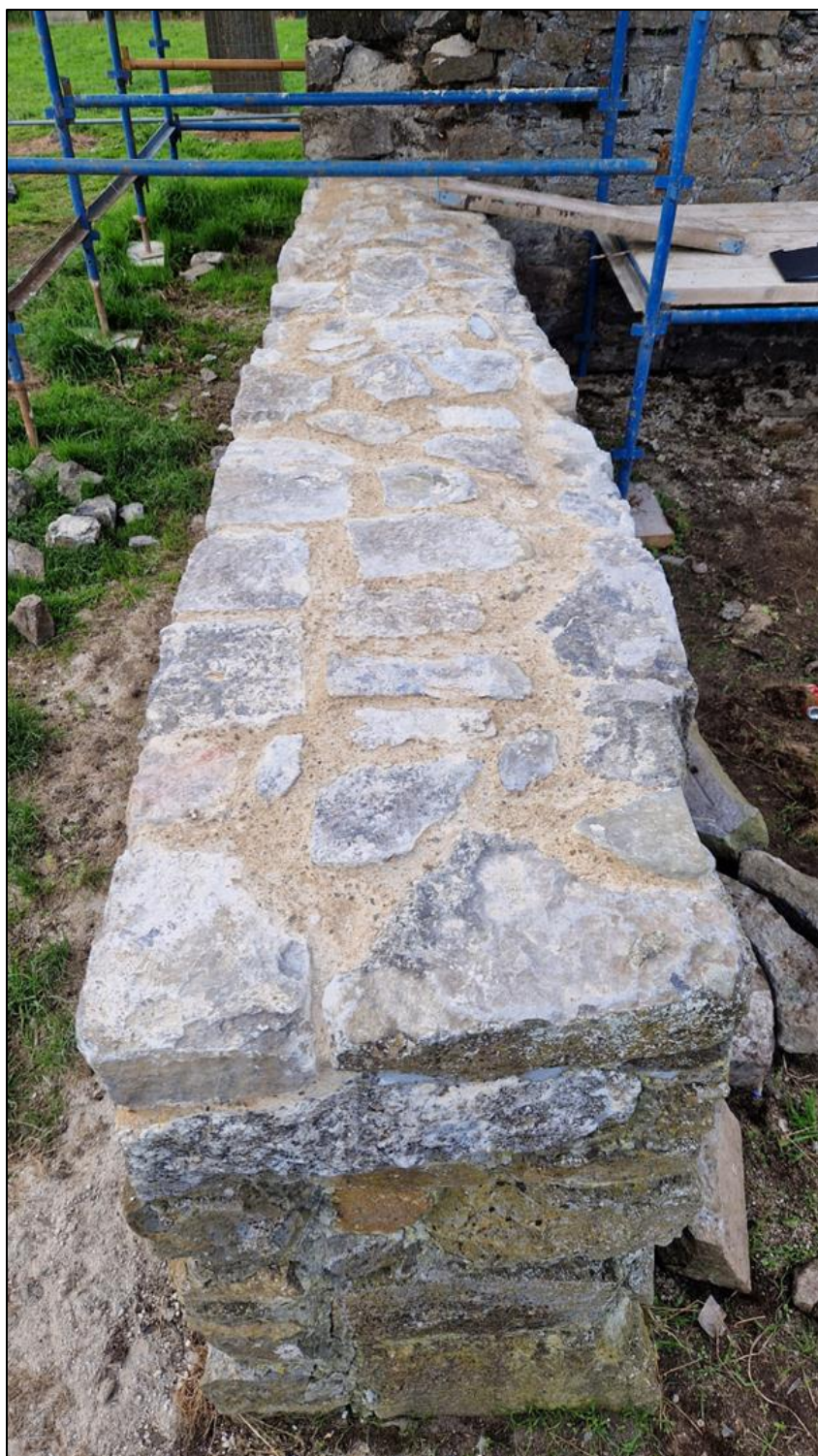
Plate 15 South wall west of entrance after flaunching
