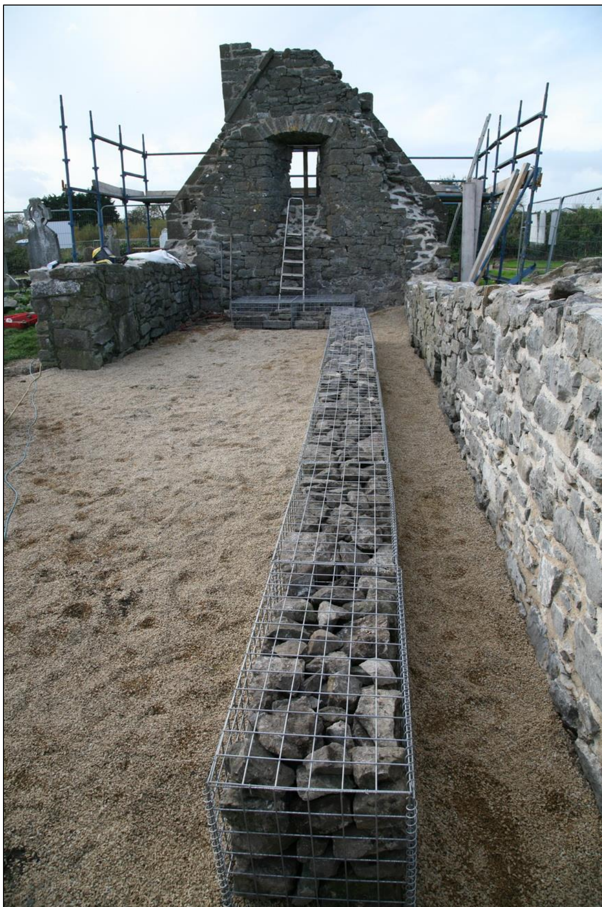
Plate 18 View of the church towards the end of conservation works
