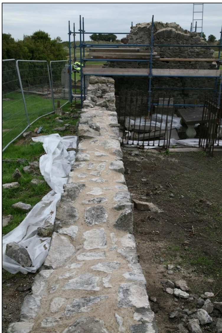
Plate 16 North wall after launching
