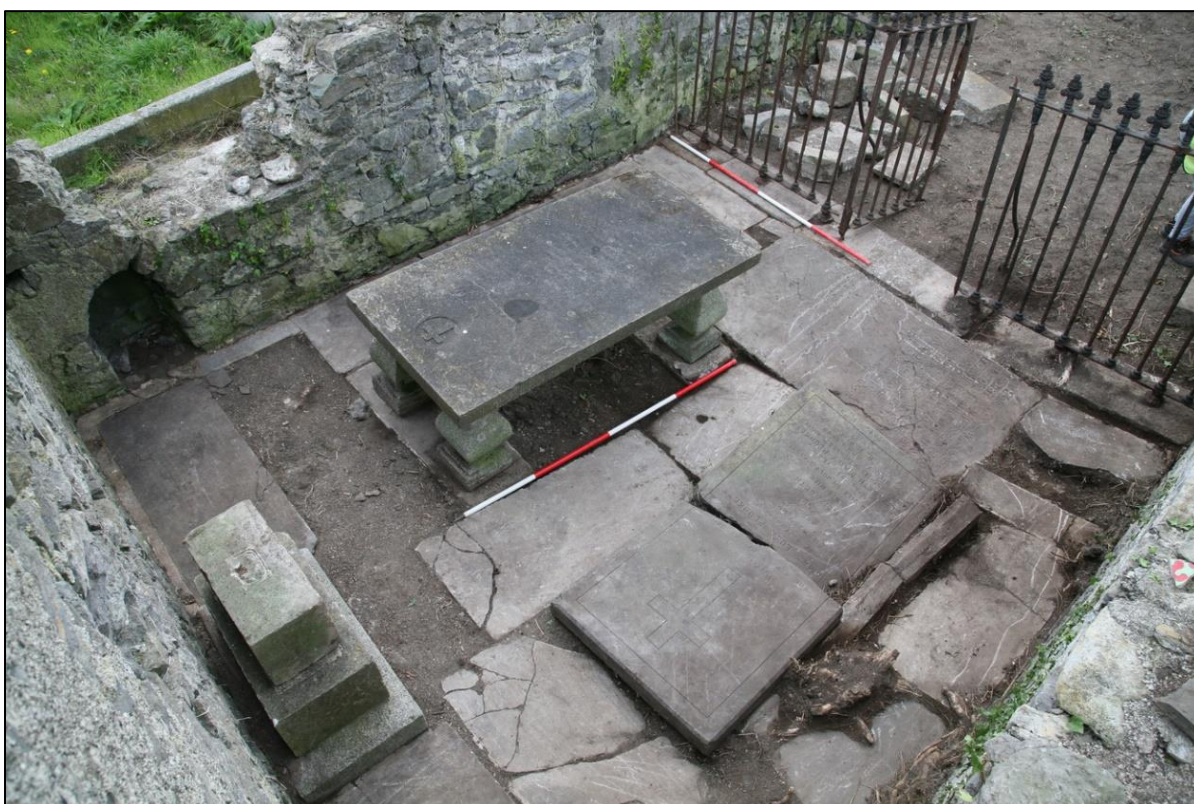
Plate 6 View of chancel area after removal of vegetation, looking southwest
