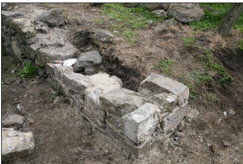
Plate 10 East entrance reveal under reconstruction
