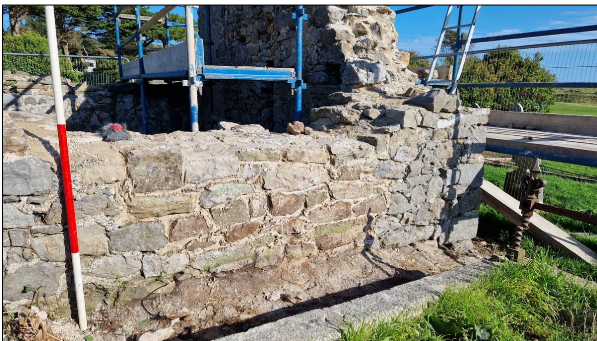
Plate 11 Reconstructed section of masonry over piscina
