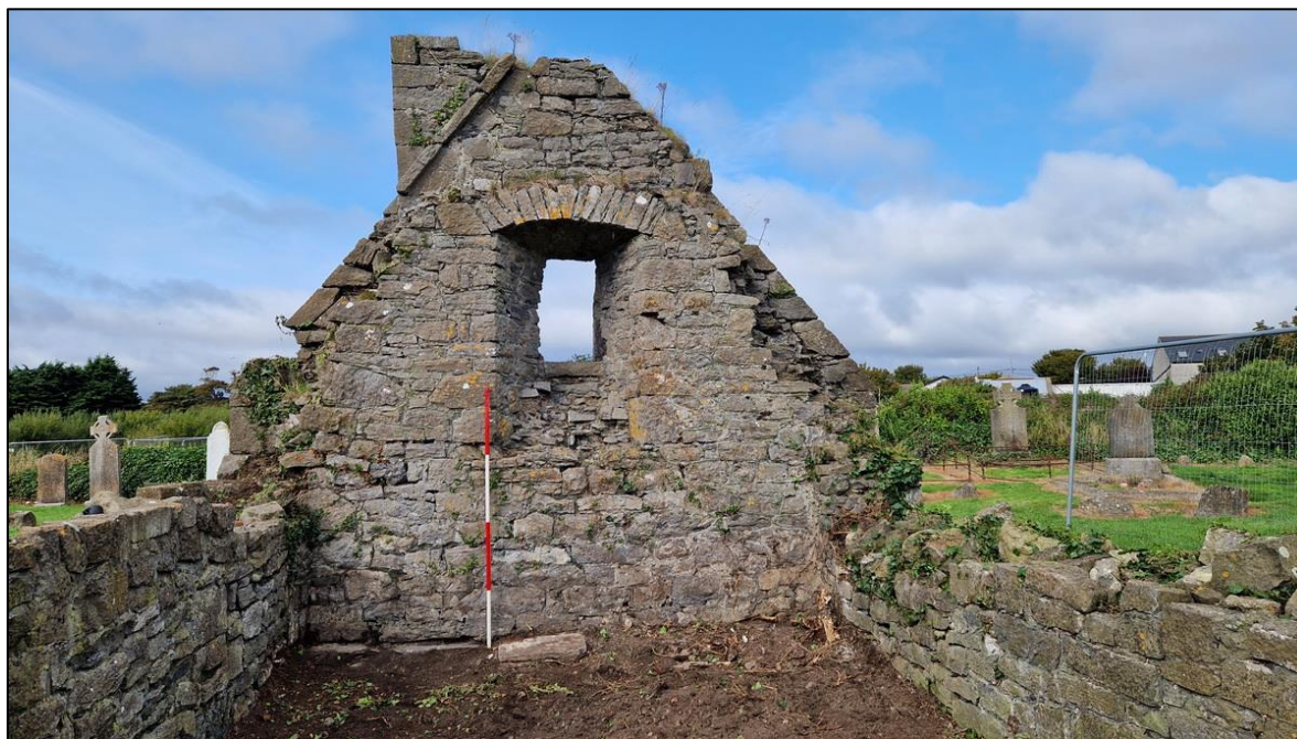
Plate 17 West gable after removal of rubble and ivy
