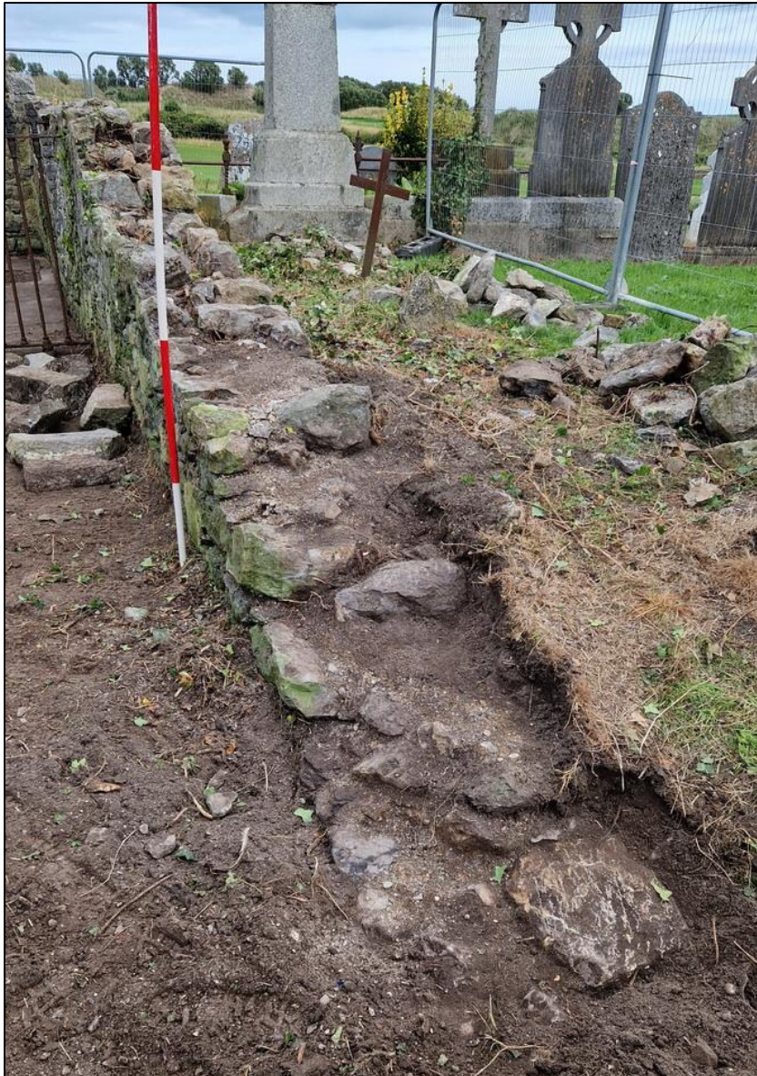
Plate 9 East entrance reveal after the removal of rubble
