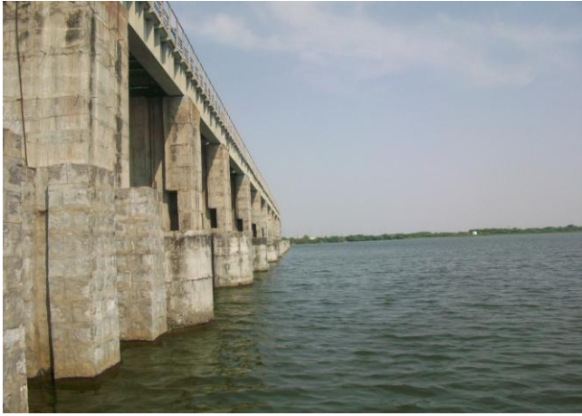
Fig. 4: Inner view of Ramanpad reservoir
