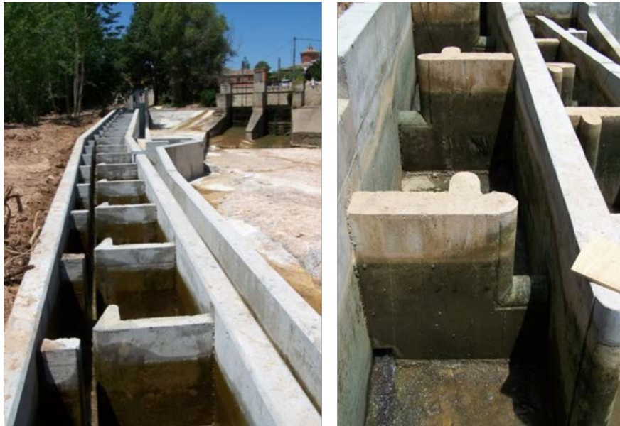
Figure 5: Test case fishways (at closed gate). Left: vertical slot fishway at Vadocondes HPP dam. Right: Submerged notch with bottom orifice fishway at Guma HPP dam
