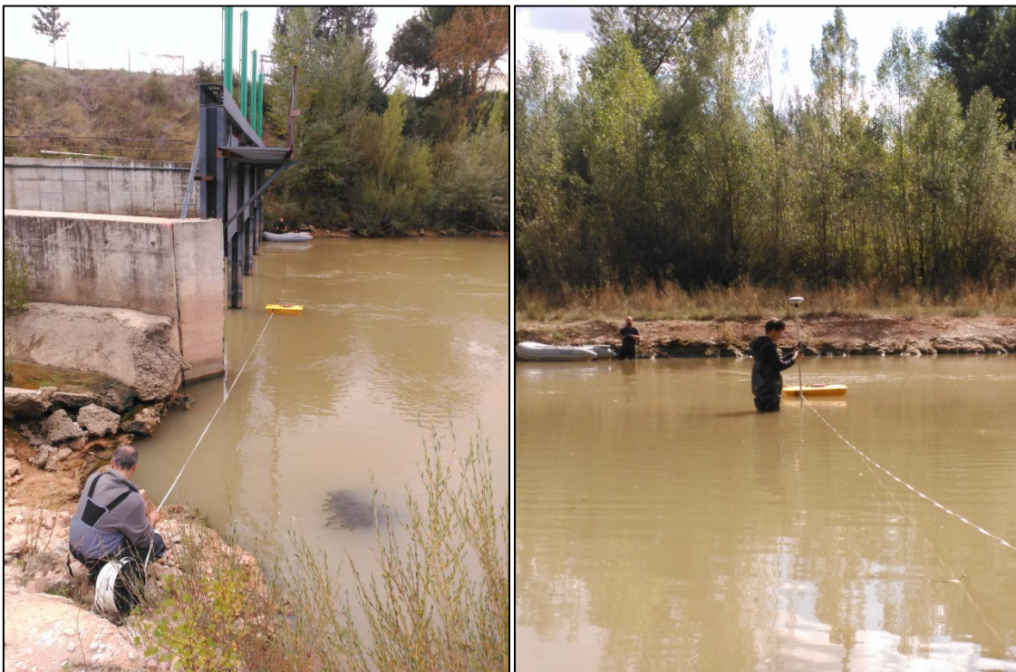
Figure 19: Hydraulic data acquisition on Guma HPP. Left: Doppler bathymetry in the turbine tailrace. Right: topographic survey of bathymetry sections
