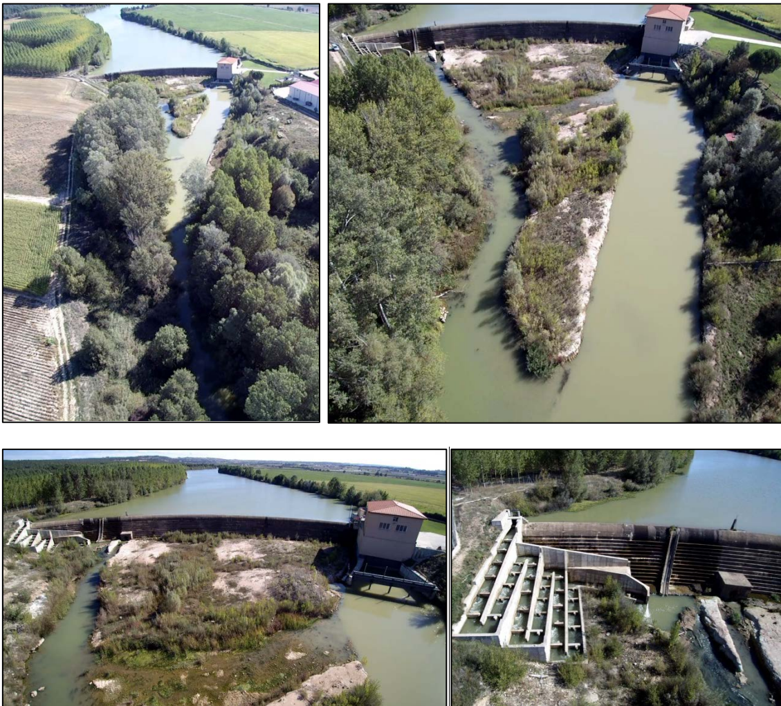
Figure 21: Photos from drone flight over Guma HPP
