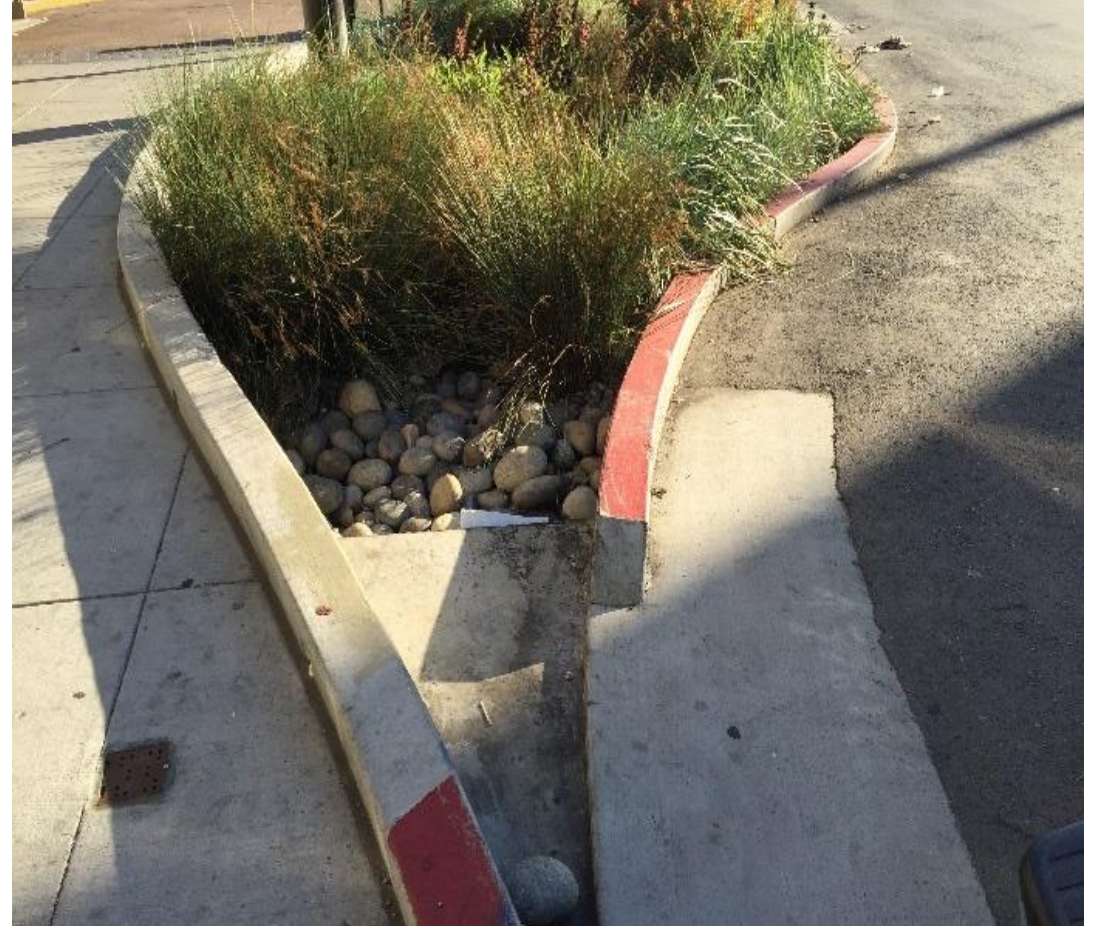
In-line design with Splash Apron and Cobbles
