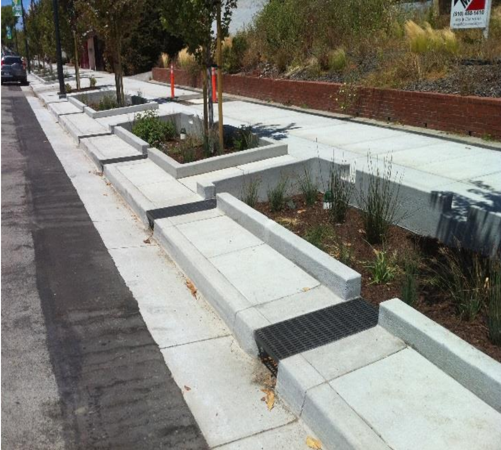
Off-line design with trench drains
