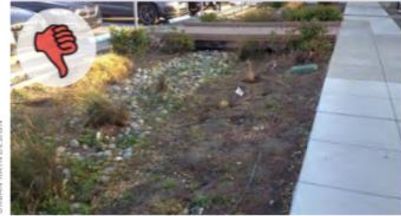
Poor, Overhaul Maintenance Routine
