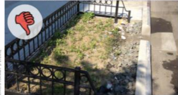
Poor, Overhaul Maintenance Routine
