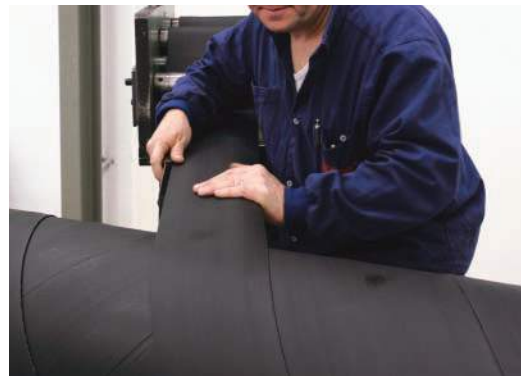
Steel cord reinforcement application
