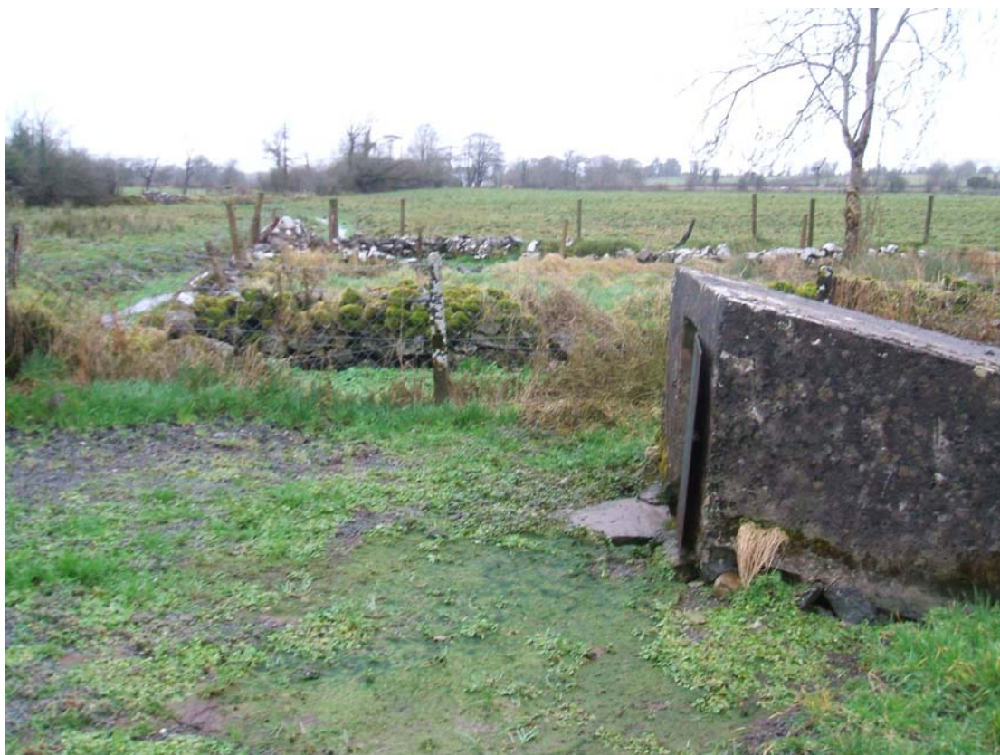
Figure 3-1. Vulnerable Spring with Inadequate Source Protection.
