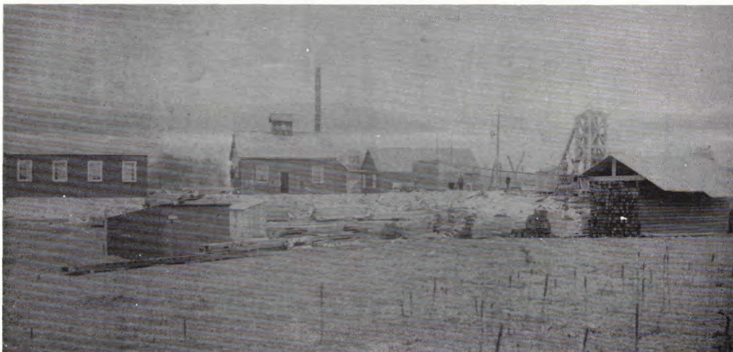
The temporary head-frame for sinking the Parker Shaft, on the right, with the engine house and machine shop to the left. This is 1891 or 1892, before flooding delayed the operation over a year. ( FMM Archives photograph. )
