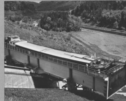
Arzwiller Water Sled Eliminates the Need for Locks
