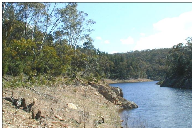
Plate 9 – Kersbrook NFR boundary with the South Para Reservoir.
