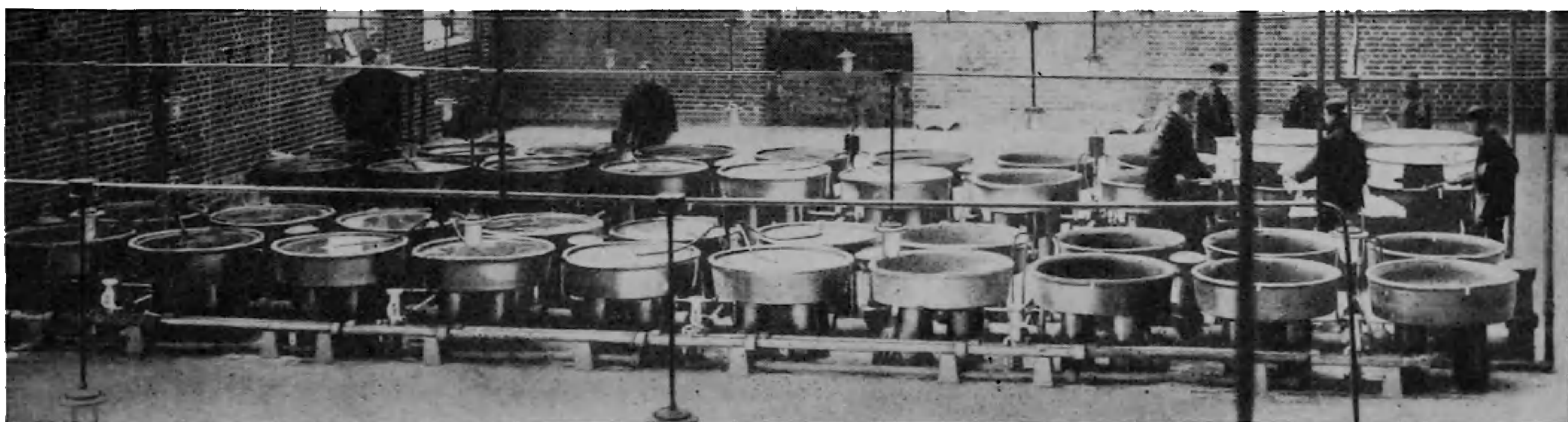
FIG. 34. View showing Arrangement of Units in Rows (from Arms and Explosives ).
