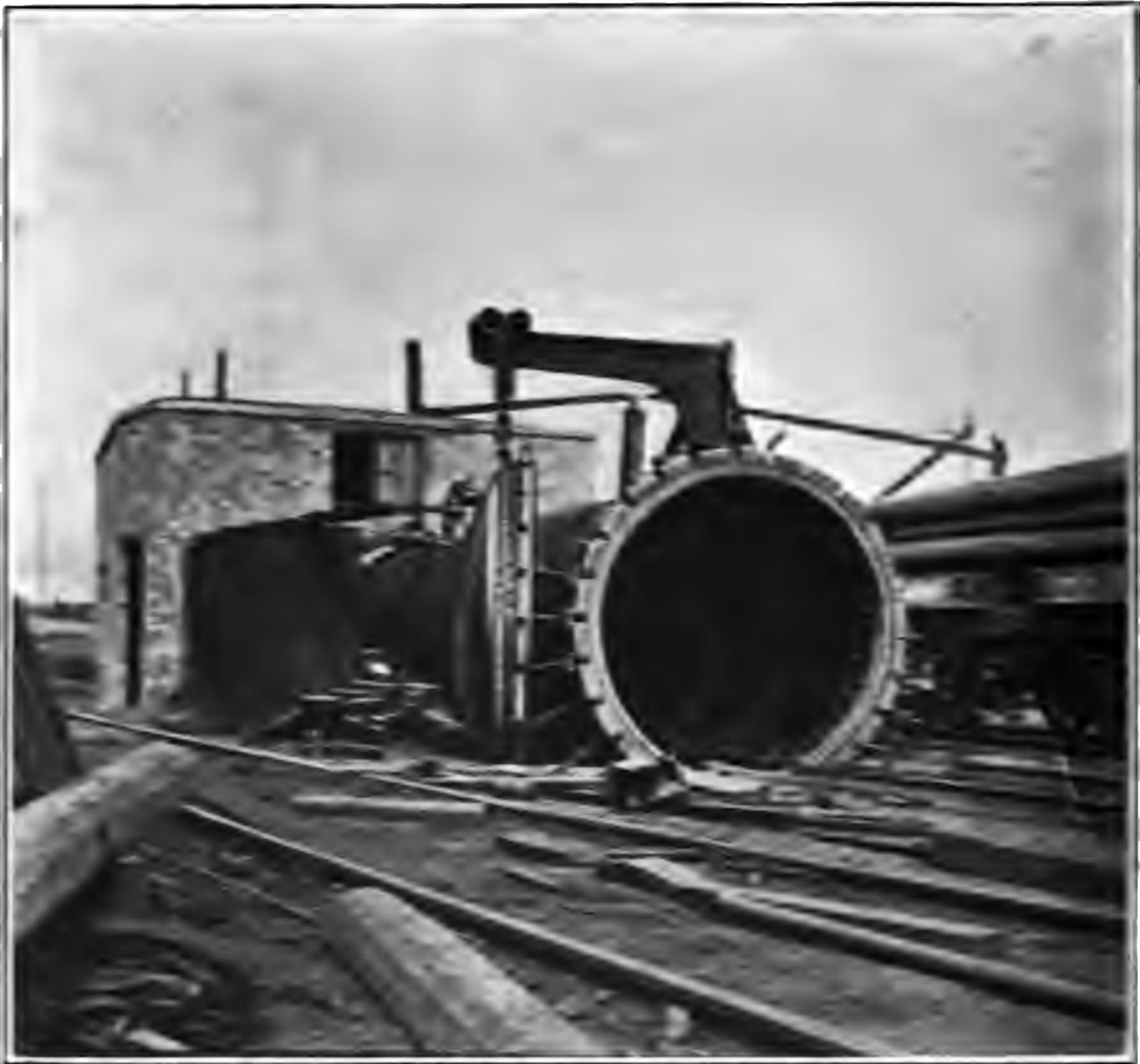
FIG. 40.—Creosoting Tank empty.
