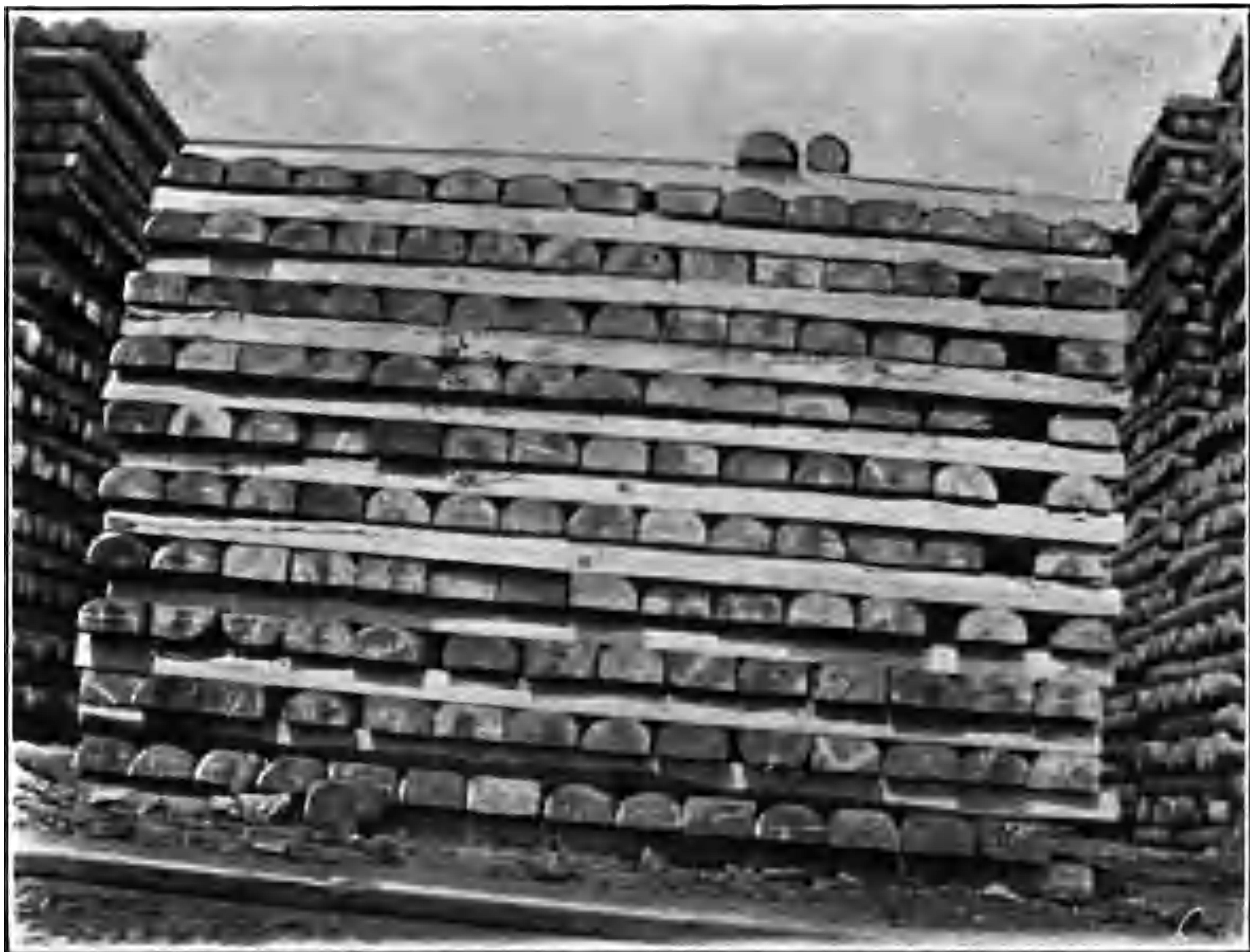
FIG. 38.—Showing Method of Stacking Sleepers for Seasoning.
