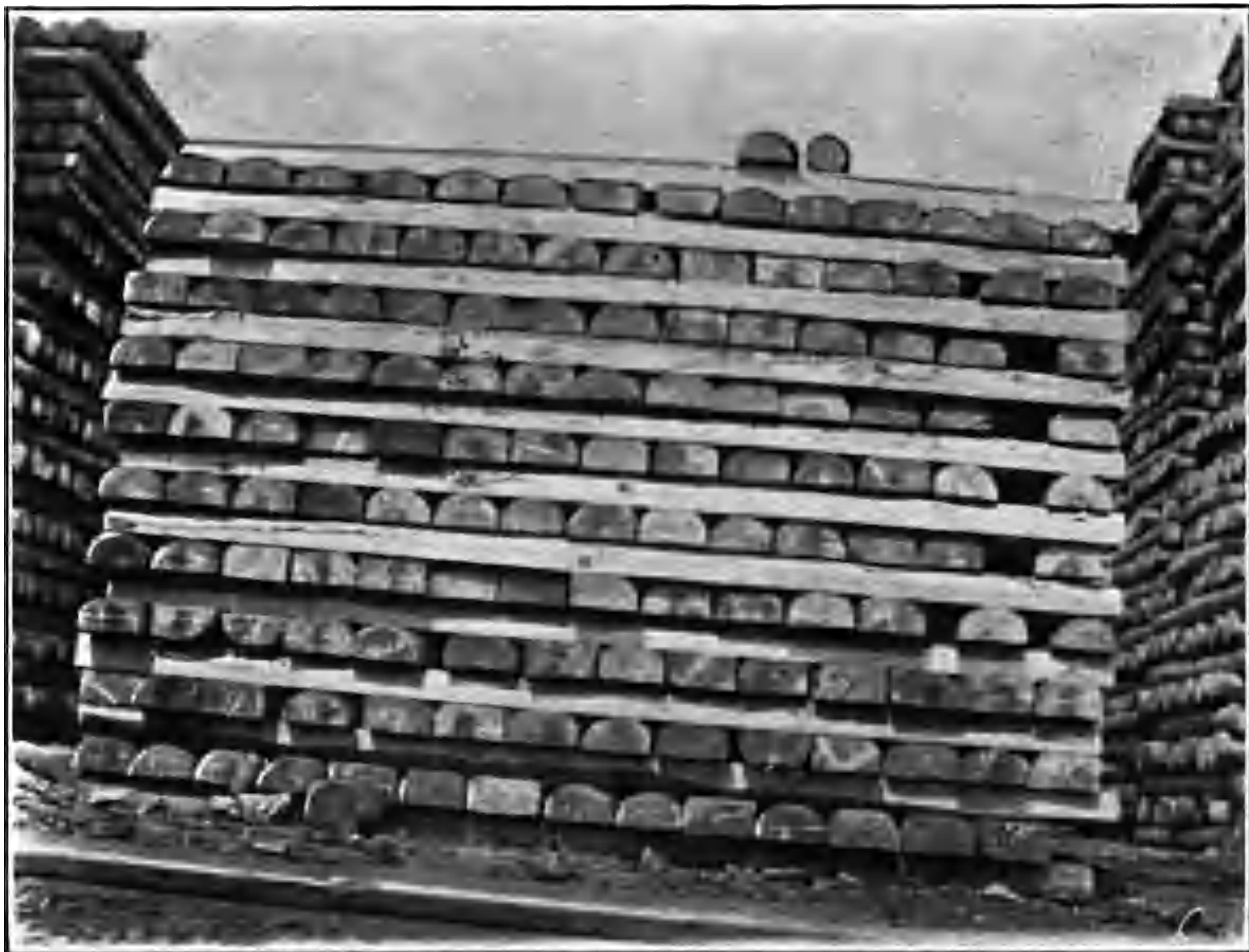
FIG. 38.—Showing Method of Stacking Sleepers for Seasoning.
