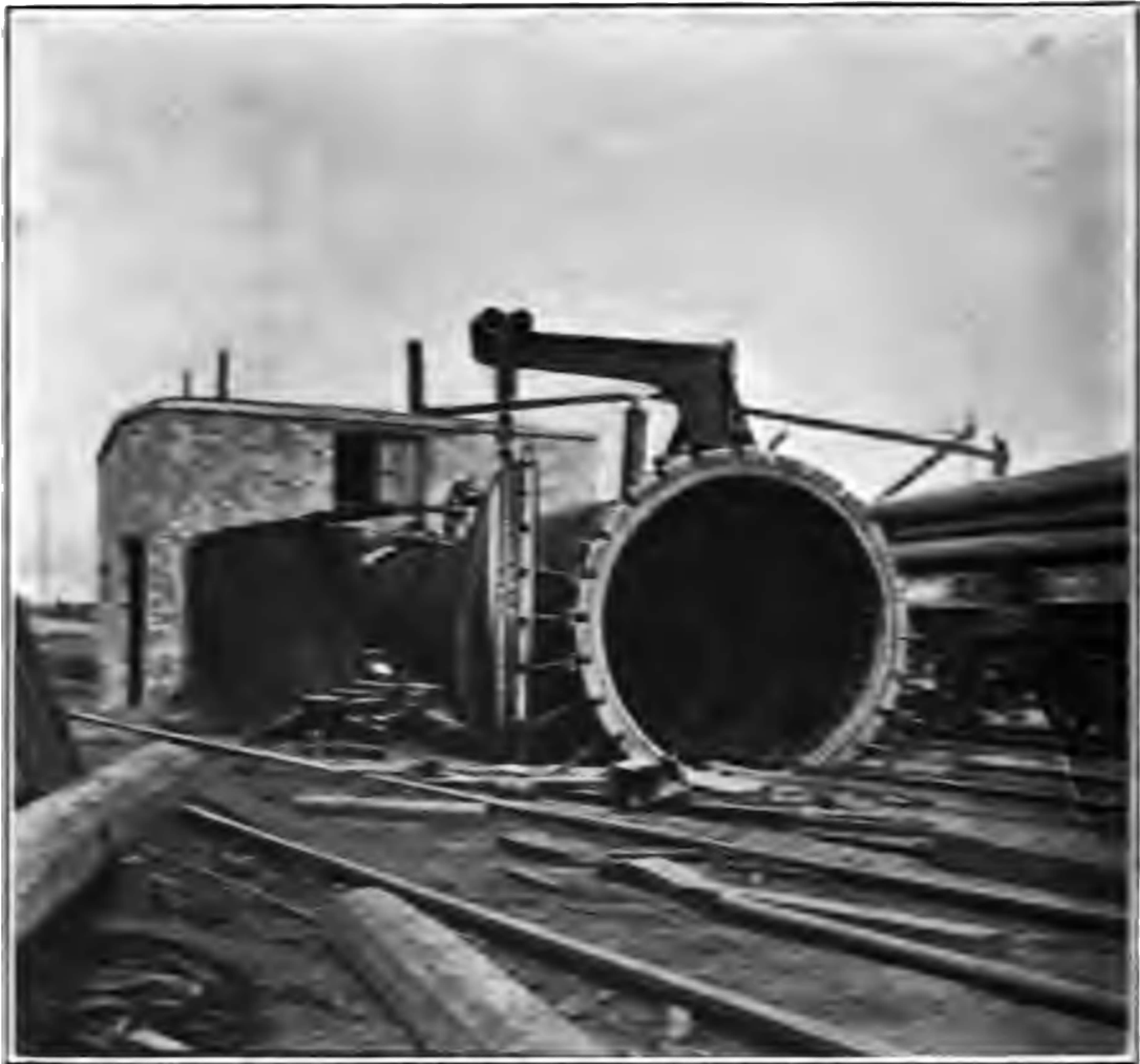
FIG. 40.—Creosoting Tank empty.
